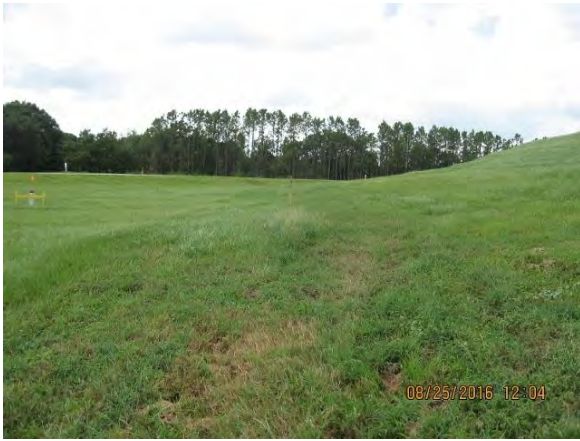
TH-67 - Berm (looking S)
