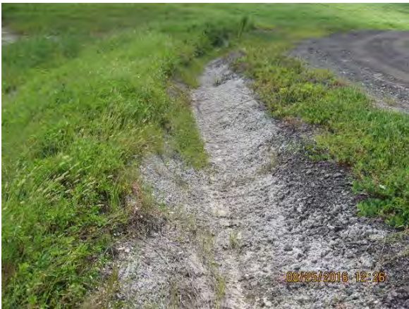
New swale for TH-71A diversion
