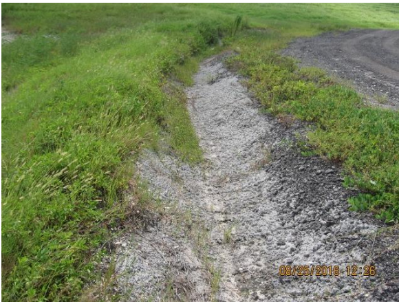
New swale for TH-71A diversion
