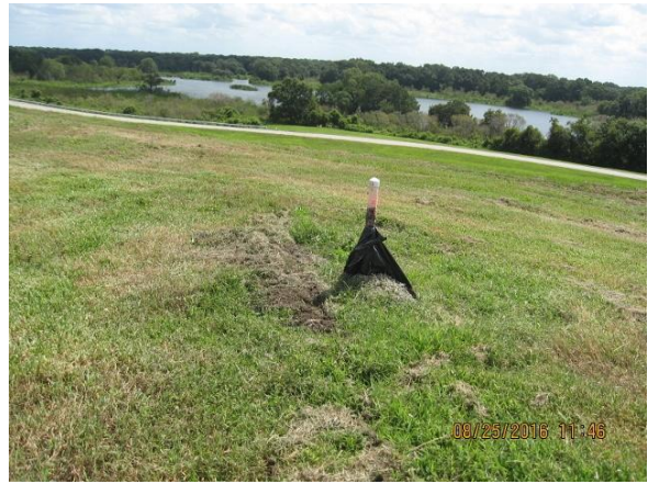
Phase II Piezometer
