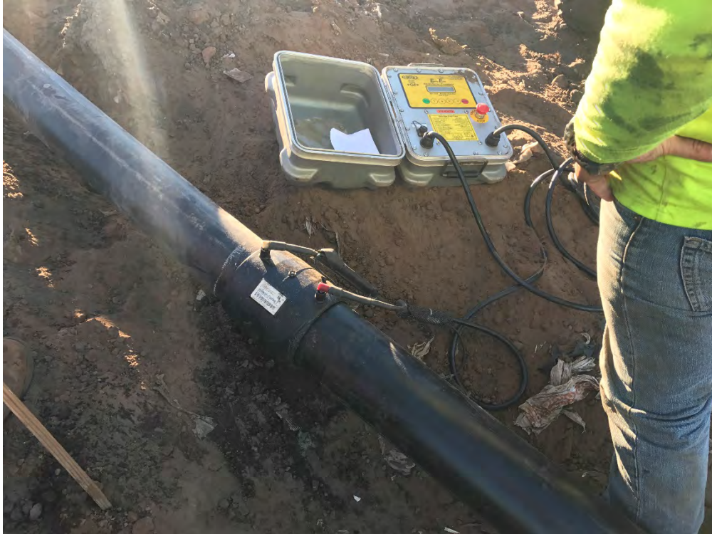
Photograph 17: Welding electrofusion coupling (typical).
