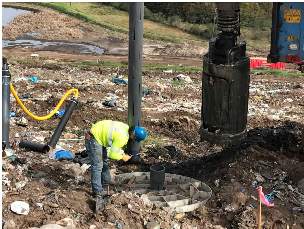
Photograph 5: Gluing slotted PVC pipes (typical).
