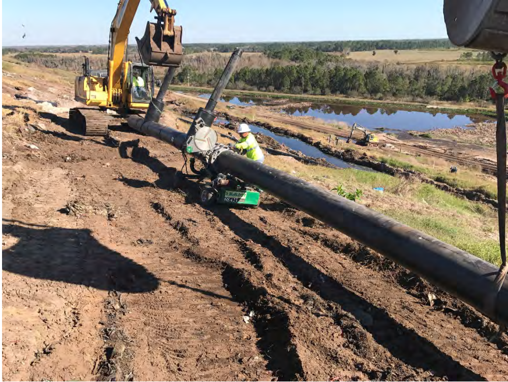
Photograph 15: Welding 18" header pipe.
