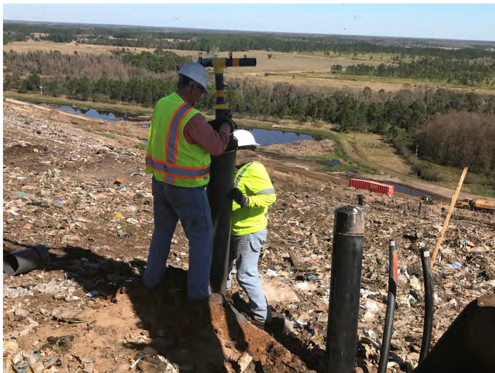
Photograph 12: Installing new wellhead (typical).
