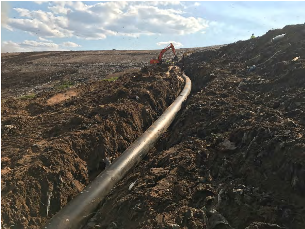
Photograph 16: 18" header pipe in trench.
