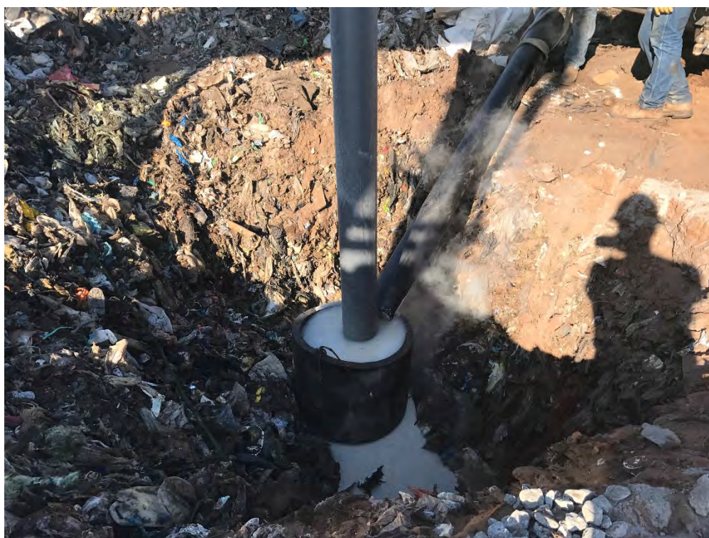
Photograph 10: Hydrating bentonite plug in encasement at JEDGW114.
