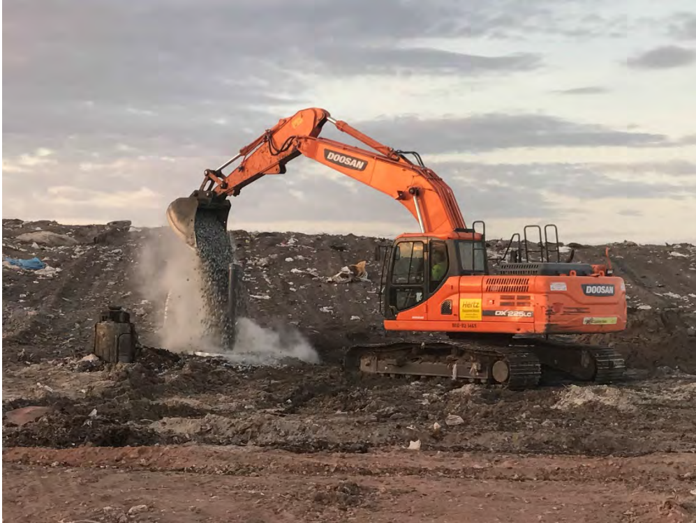
Photograph 7: Backfilling extraction well with approved stone (typical).
