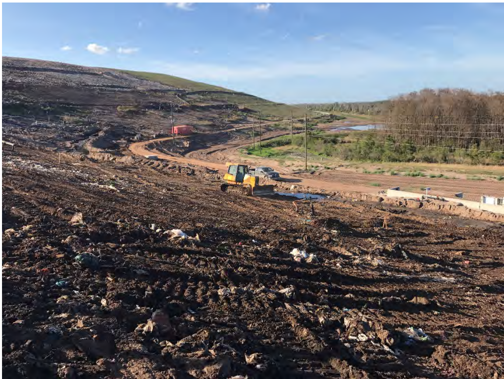
Photograph 24: Regrading slopes with dozer (typical).
