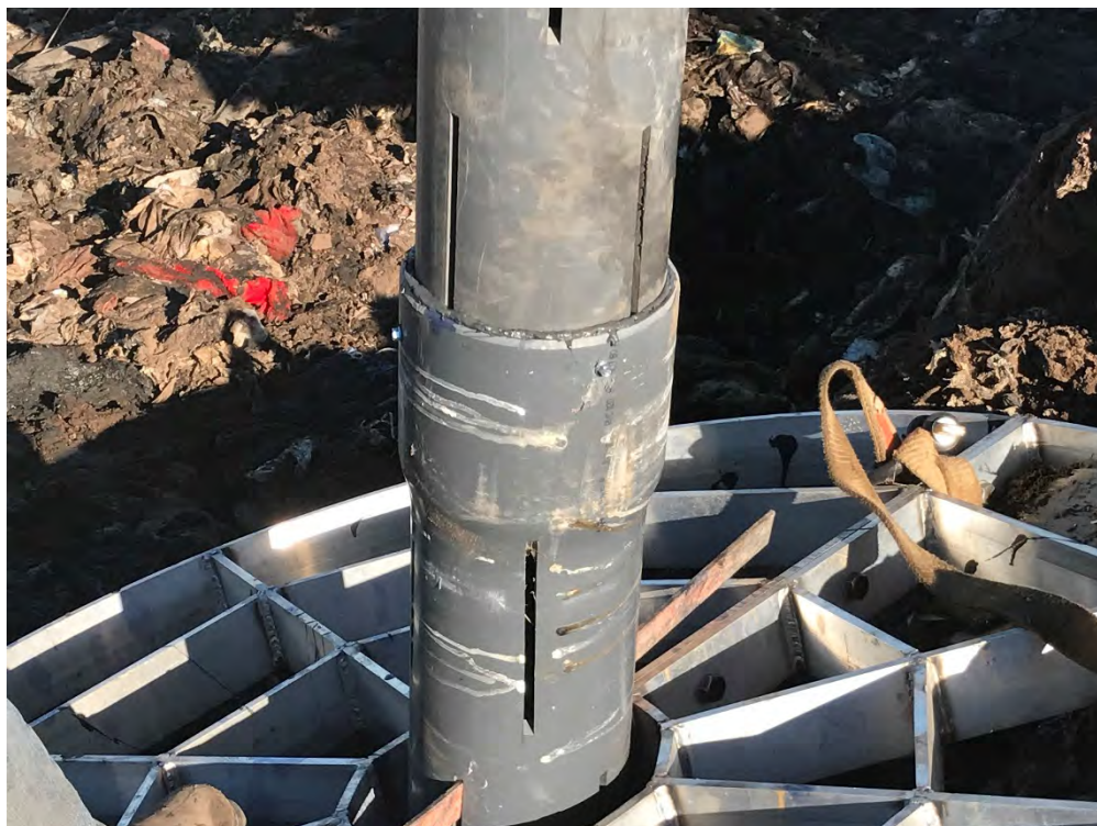
Photograph 6: Lag bolted joints to provide additional support (typical).
