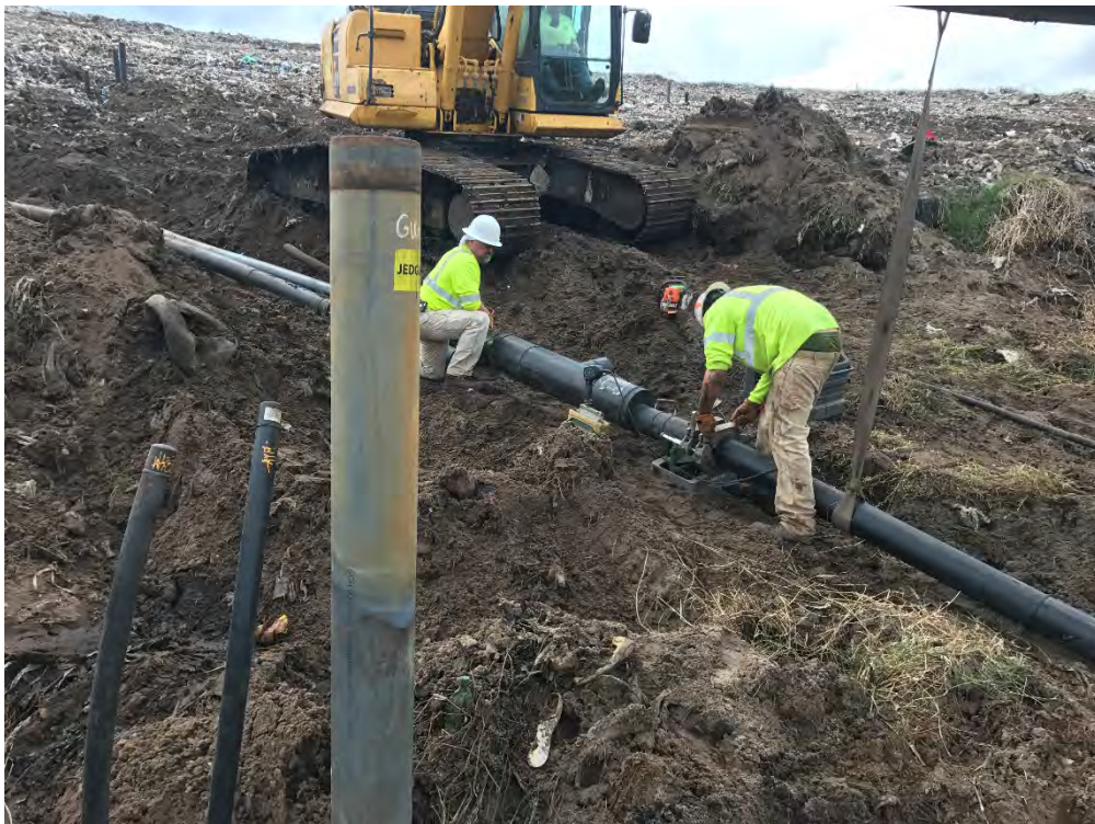
Photograph 18: Welding 8" lateral.
