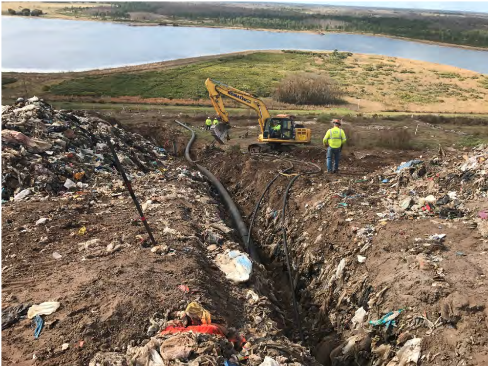
Photograph 20: Installing lateral pipe in trench with air supply line and forcemain.
