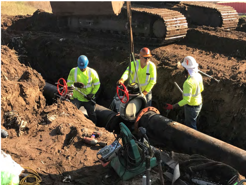
Photograph 22: Installing valves on header pipe.
