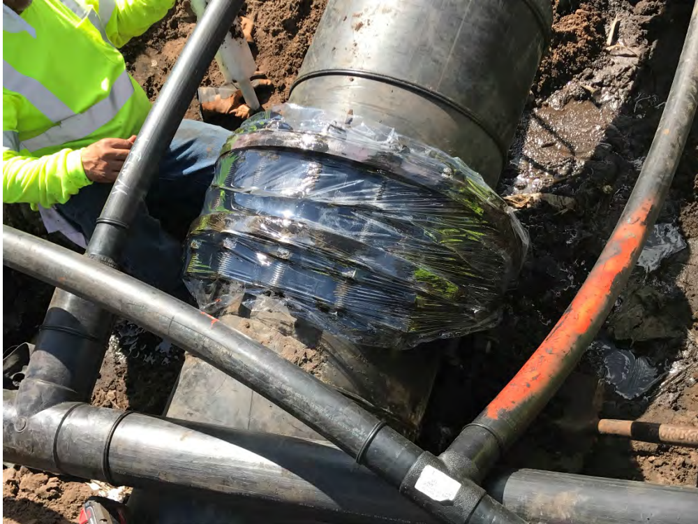
Photograph 21: Flange bolts wrapped with 10 mil plastic and taped to pipe.
