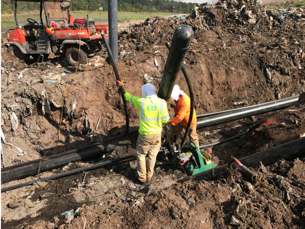
Photograph 19: Welding 2" air and 2" forcemain.
