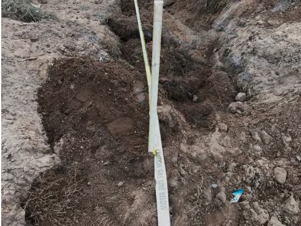
Photograph 23: Backfilling trench. Caution tape applied and survey posts every 50' and at points of interest (typical).
