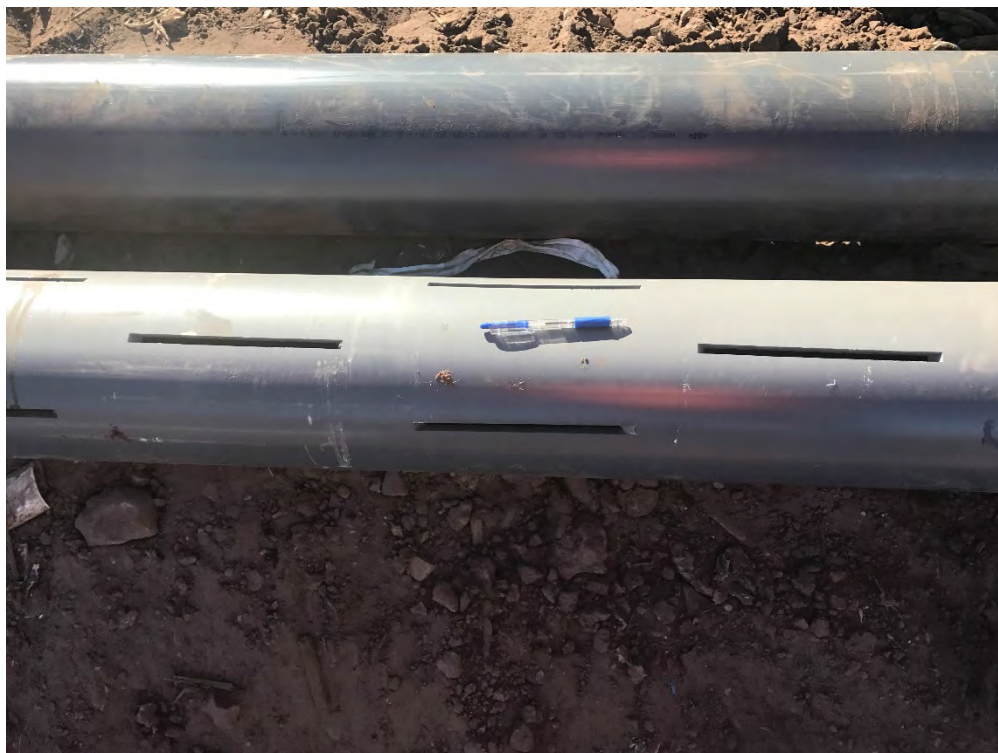
Photograph 1: 8" SCH 80 slotted and solid PVC pipes.
