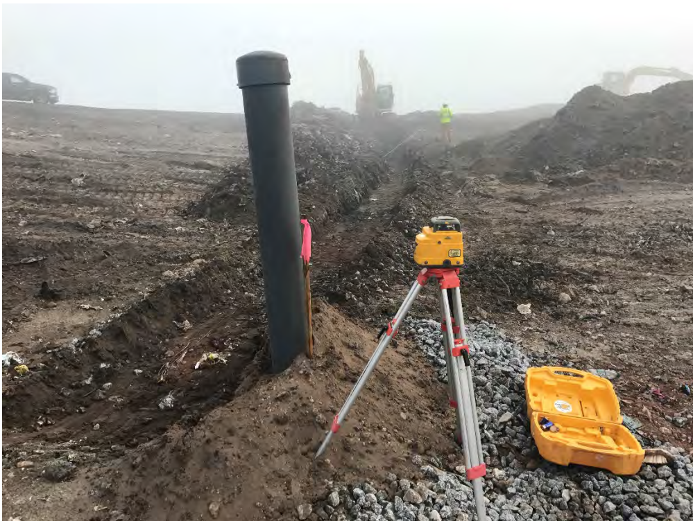
Photograph 14: Checking trench slope while excavating.
