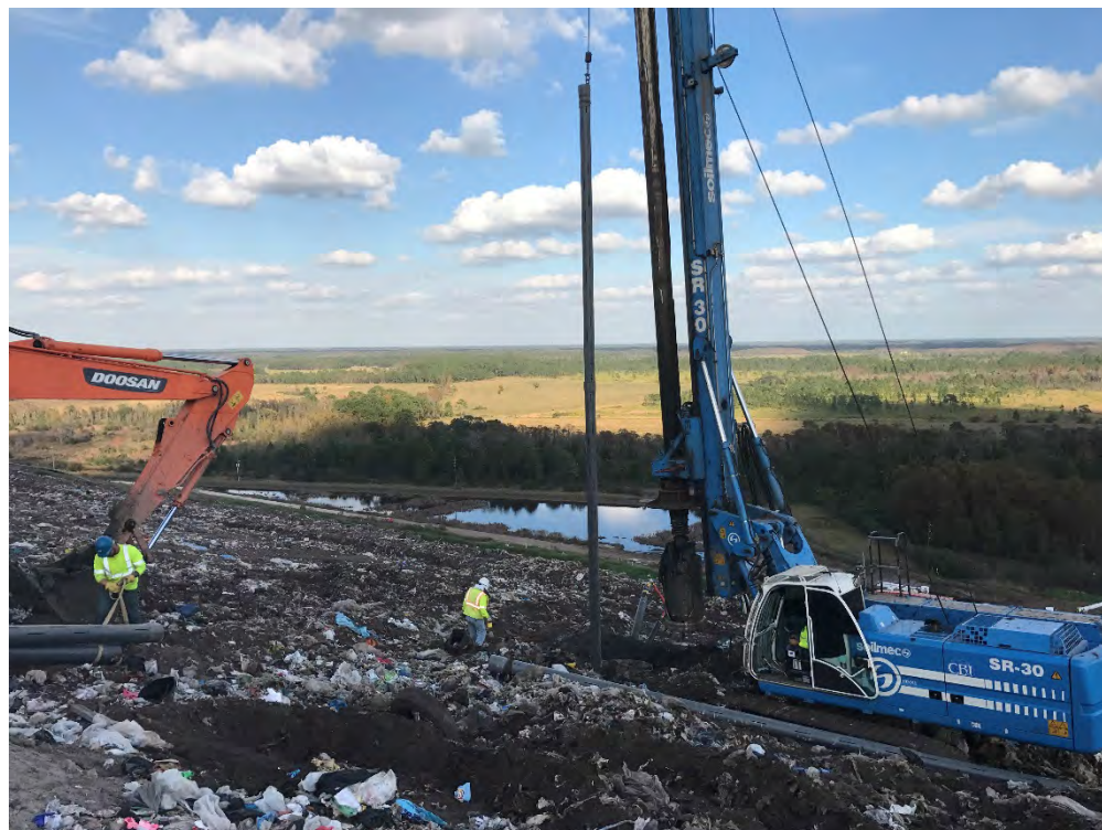
Photograph 4: Setting gas well screen (typical).
