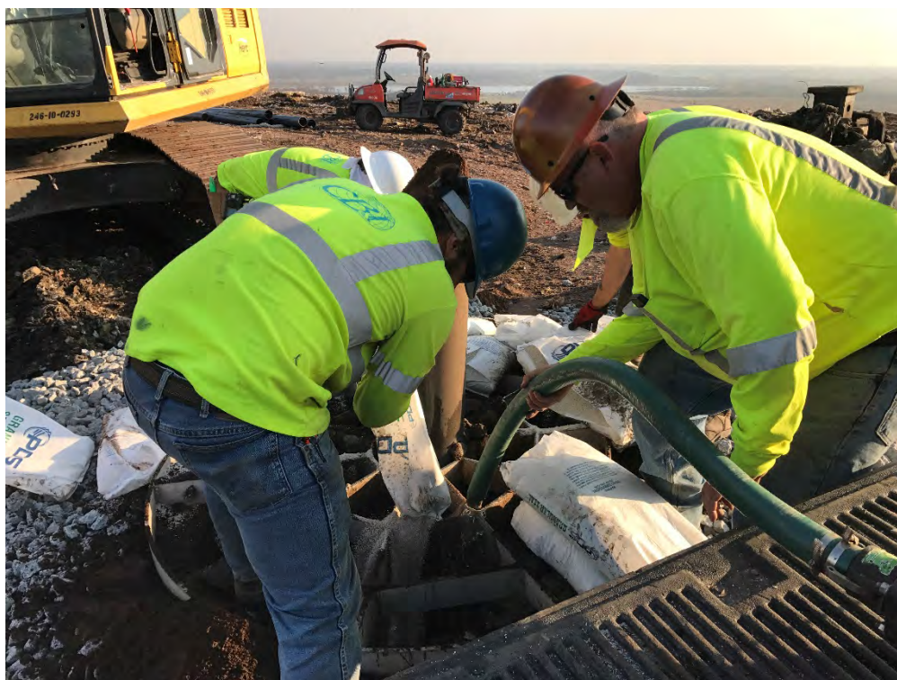
Photograph 9: Hydrating bentonite plug at extraction well (typical).
