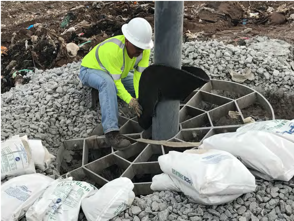
Photograph 8: Installing geogring (typical).
