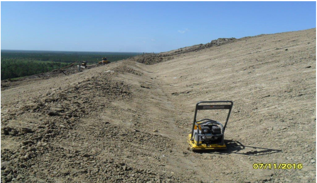
Compacting Clay at Terrace 9 within Unit 87 (Facing Southerly) (July 2016)
