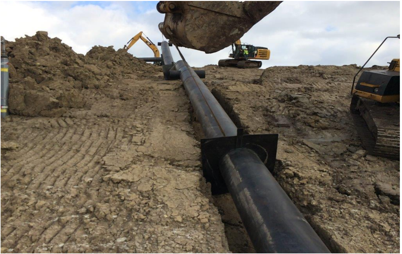
Placement of Downcomer D-52 (facing Easterly) (December 2016)
