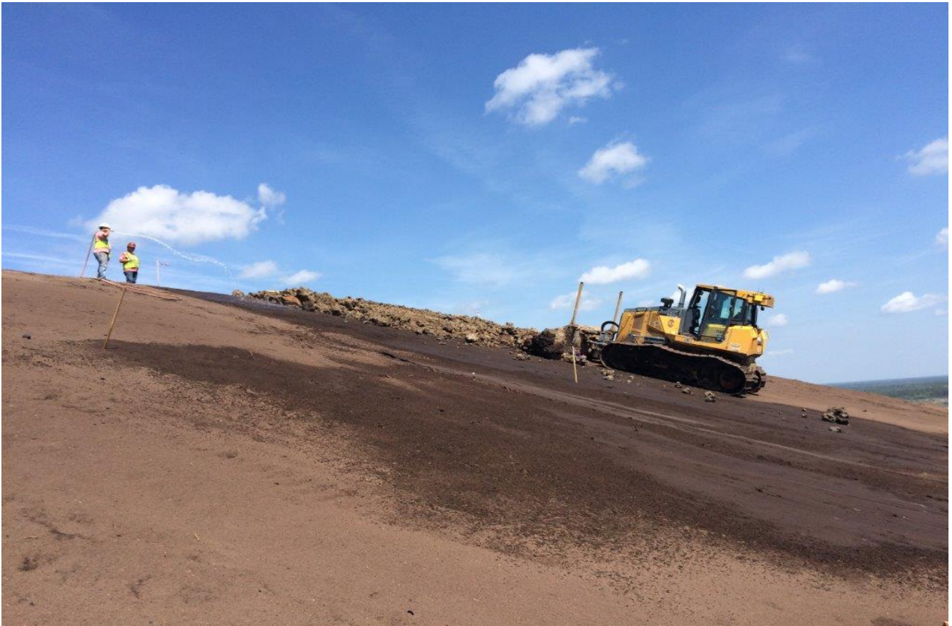
Placing Clay for Clay Test Strip (Facing Northerly) (April 2016)
