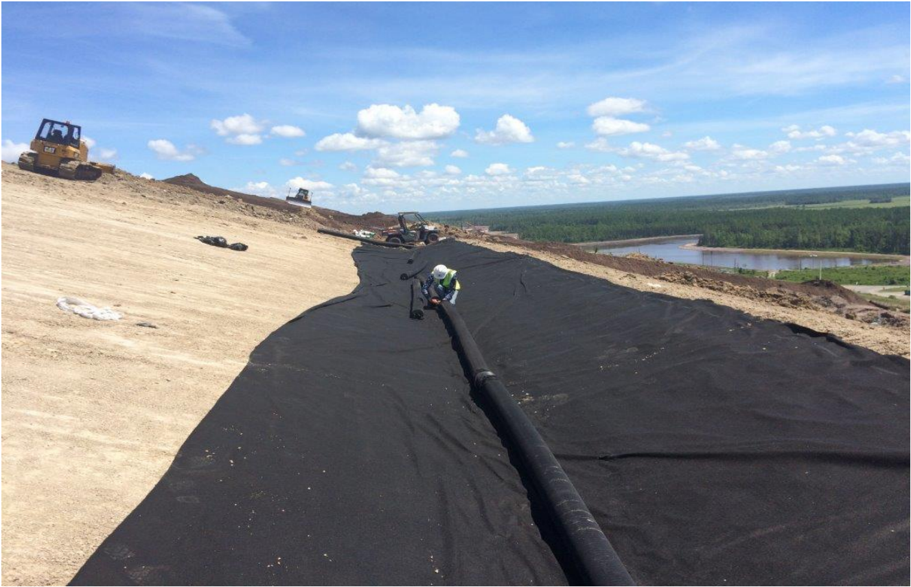
Grading underdrain pipe Terrace 9 Unit 87 (Facing Northerly) (July 2016)
