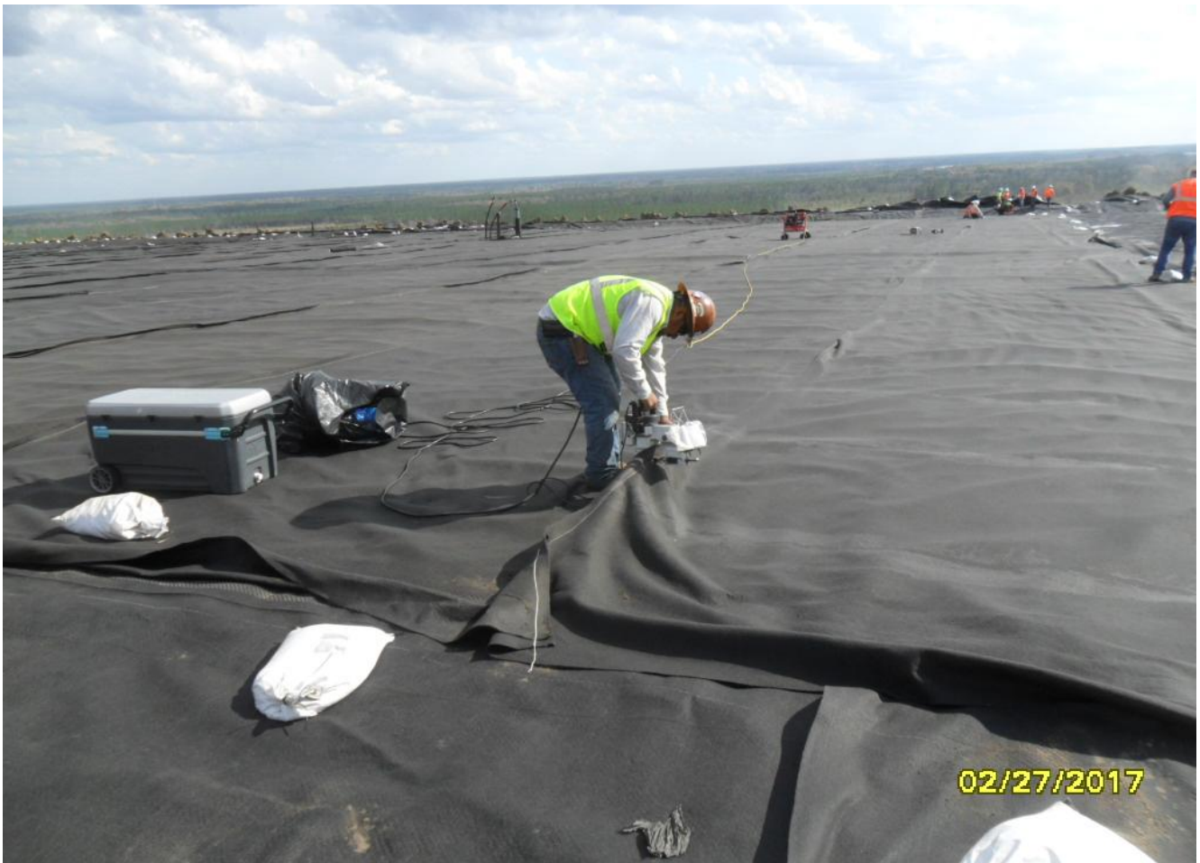
Sewing geotextile at top of hill (facing Easterly) (February 2017)
