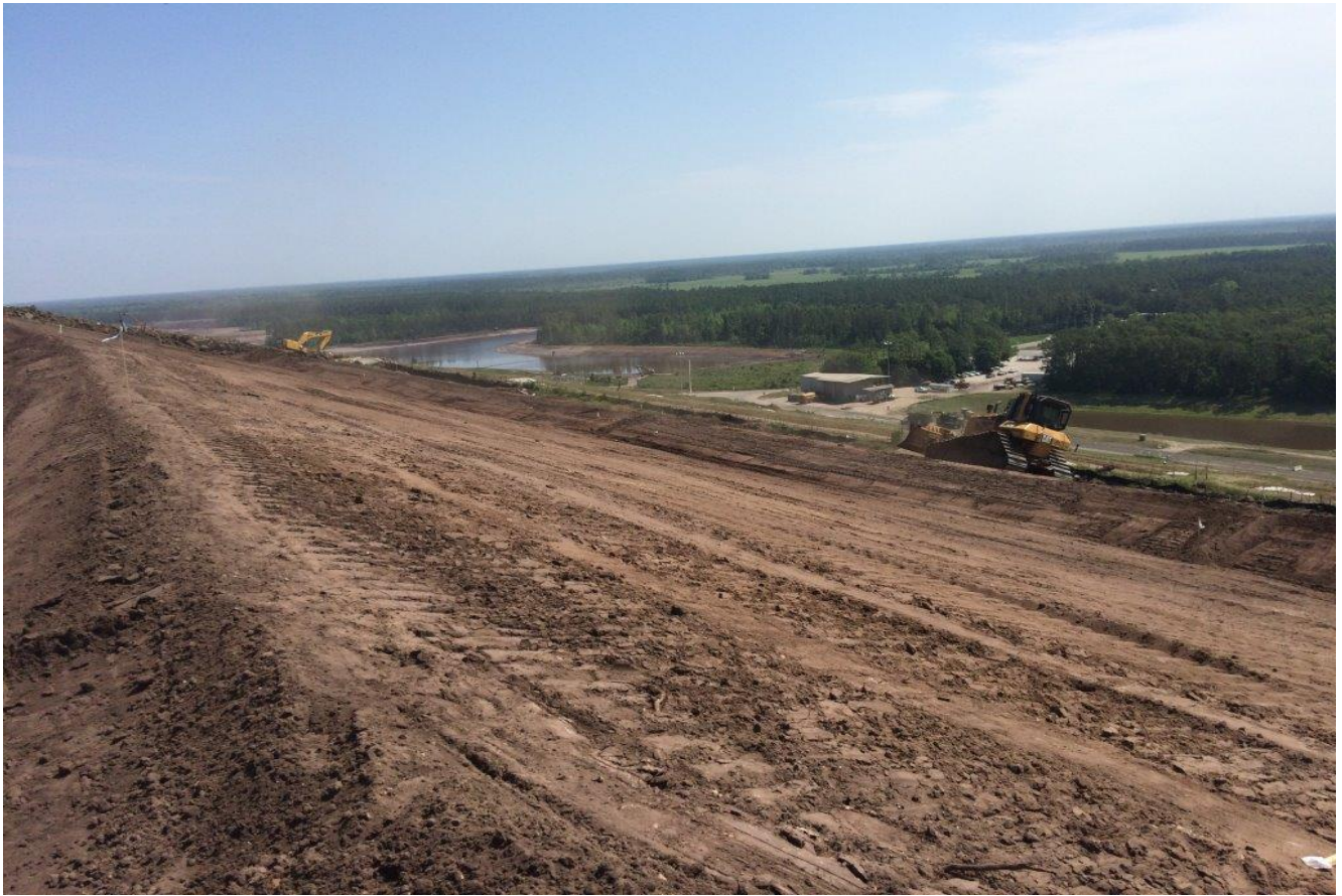
Initial Cover grading by TRLI – Units 86 and 87 (Facing Northeasterly) (May 2016)
