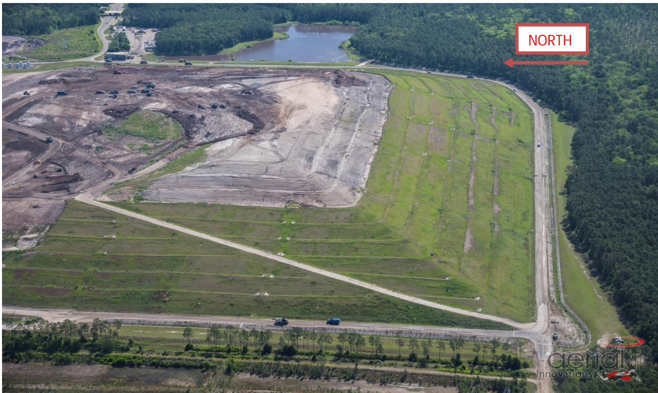
Start of Construction - Aerial Photograph - Trail Ridge Landfill (April 2016)
