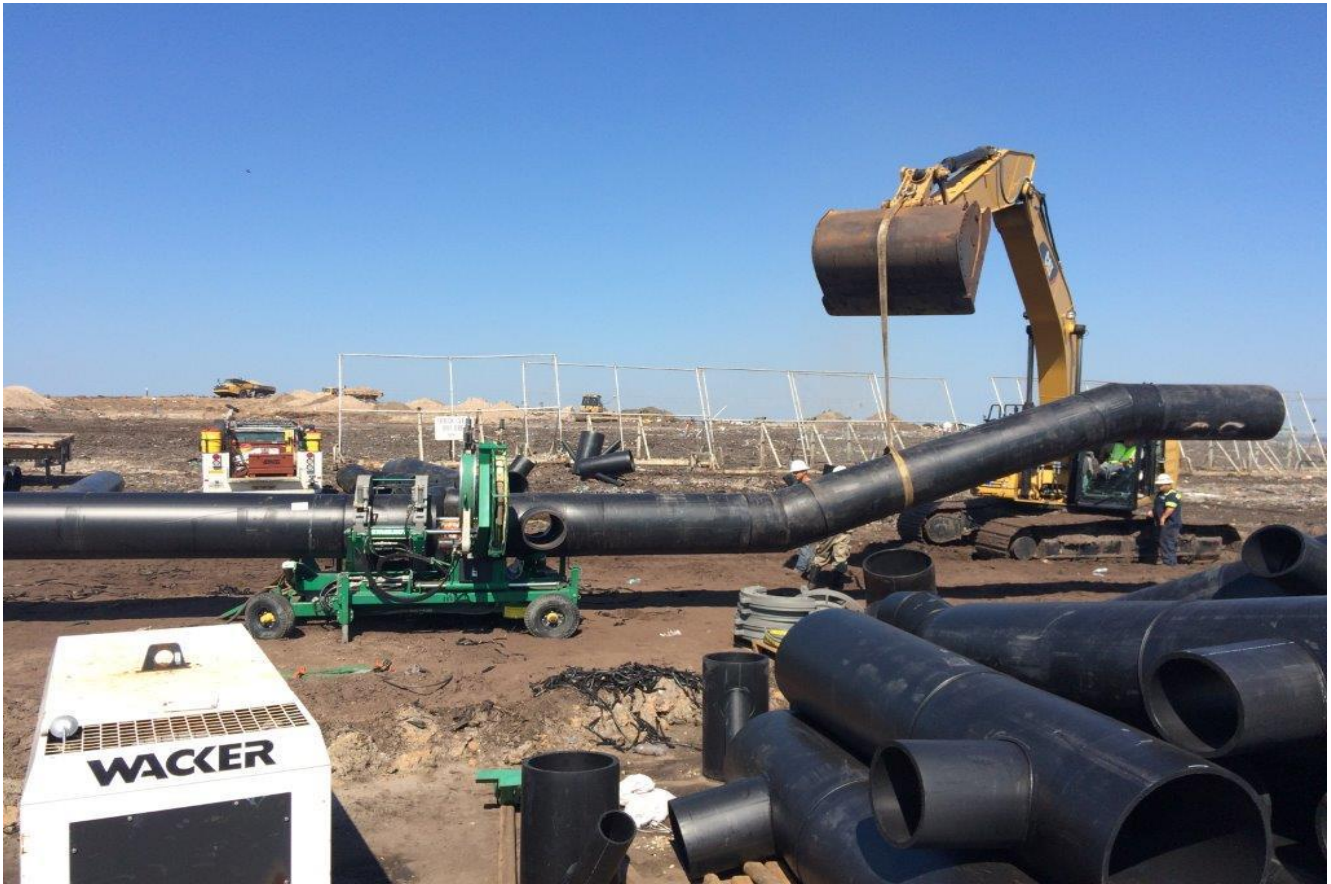
Welding Downcomer D-24 (top of the hill) (facing Southerly) (September 2016)
