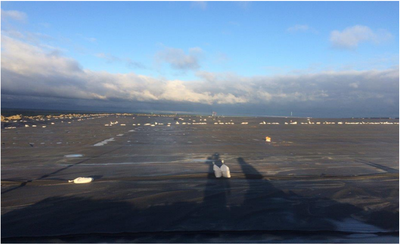
Liner deployment top of hill (westerly side) (facing Westerly) (March 2017)
