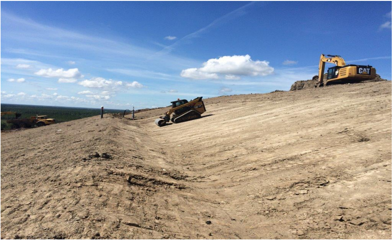
Grading and Smoothing Clay at Terrace 9 within Unit 87 (Facing Southerly) (July 2016)
