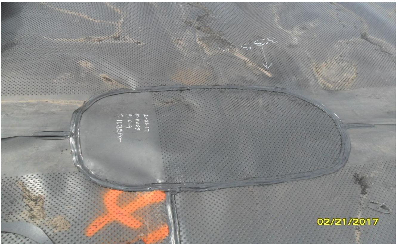
Liner repair at top of hill (easterly side) (February 2017)
