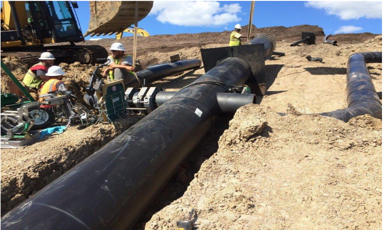
Installation of sidedrains Downcomer D-38 (facing Northerly) (October 2016)
