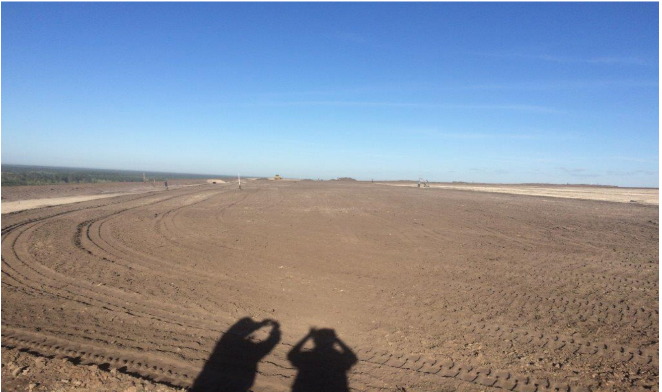
Graded top soil top of hill (facing Westerly) (April 2017)
