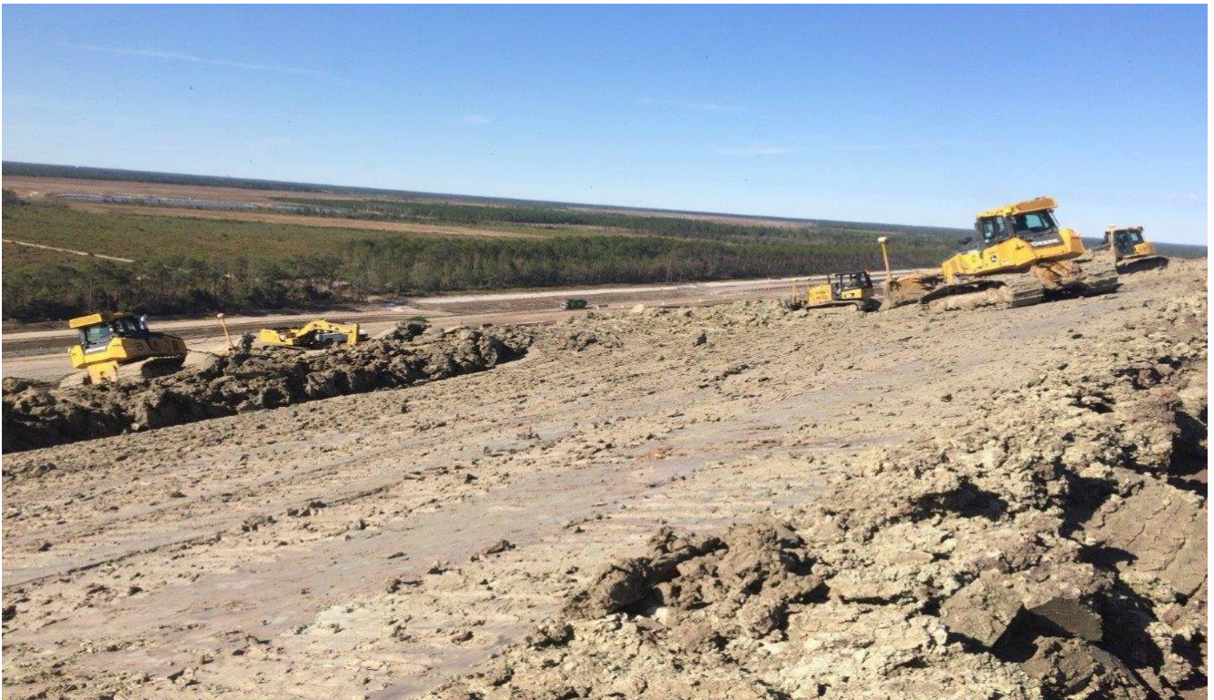
Grading clay Units 106 – 108 (facing Northerly) (December 2016)
