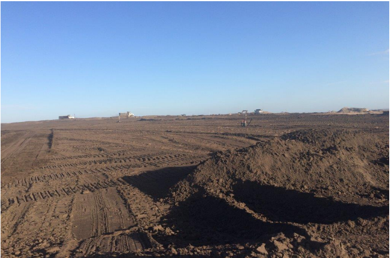
Top soil placed over geomembrane top of hill (facing Northerly) (March 2017)
