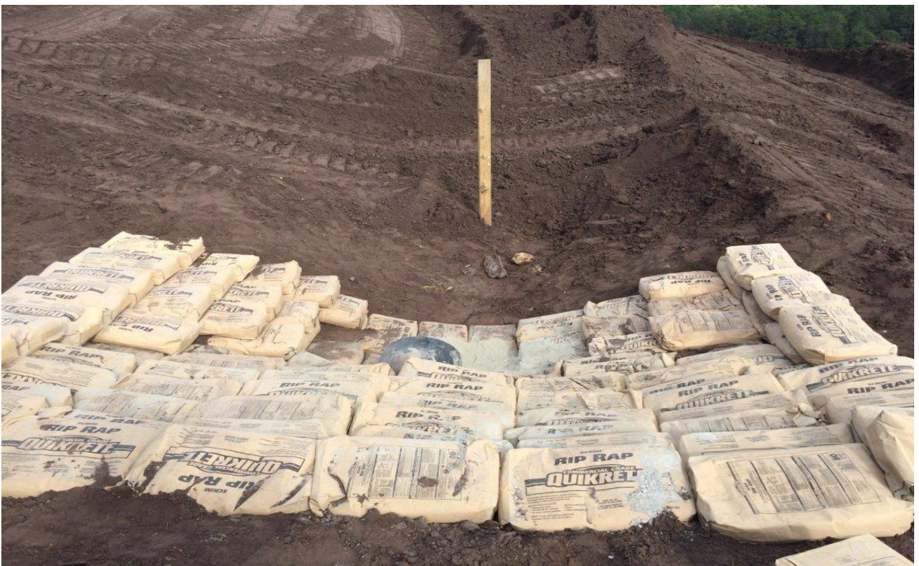
Rip Rap installation for sidedrains for Downcomer D-38 (facing Easterly) (October 2016)
