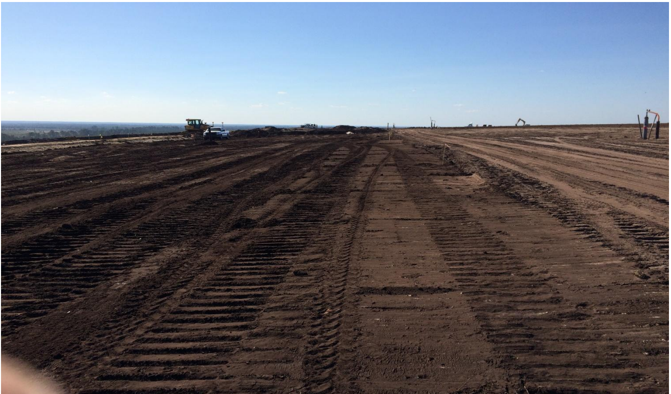
Balancing and grading behind Terrace 10 at top of hill (facing Southerly) (January 2017)
