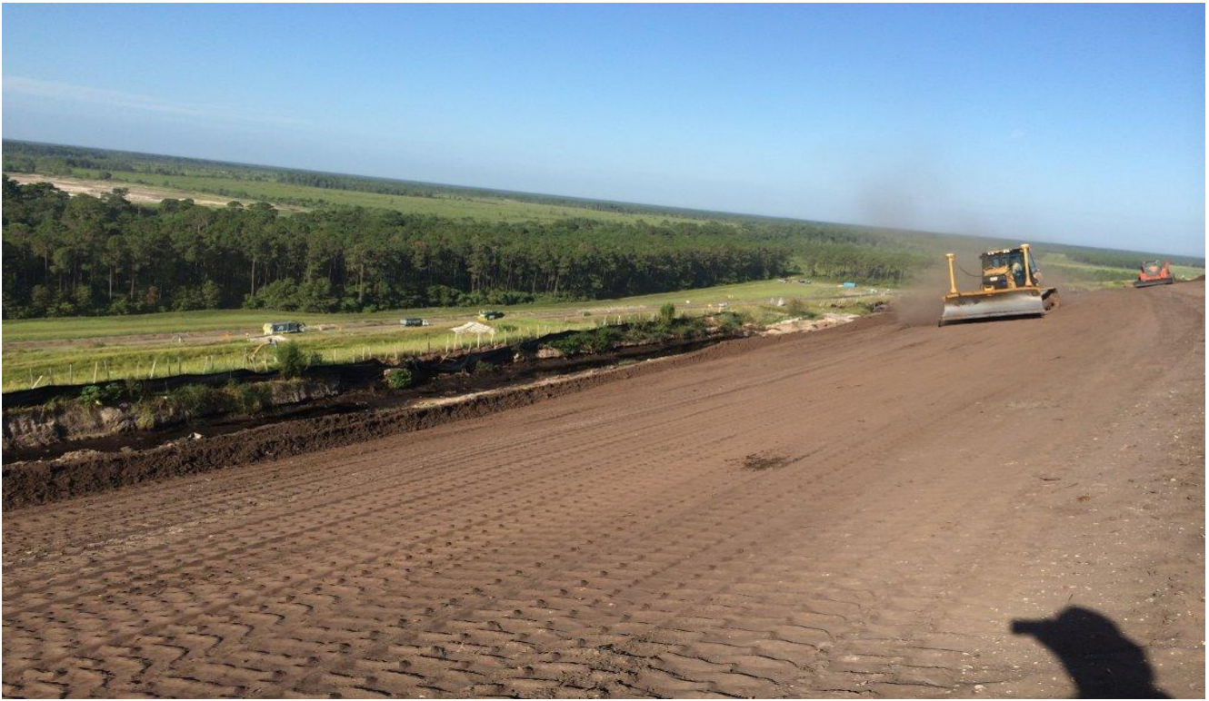
TRLI grading initial cover Unit 91 (Facing Westerly) (July 2016)
