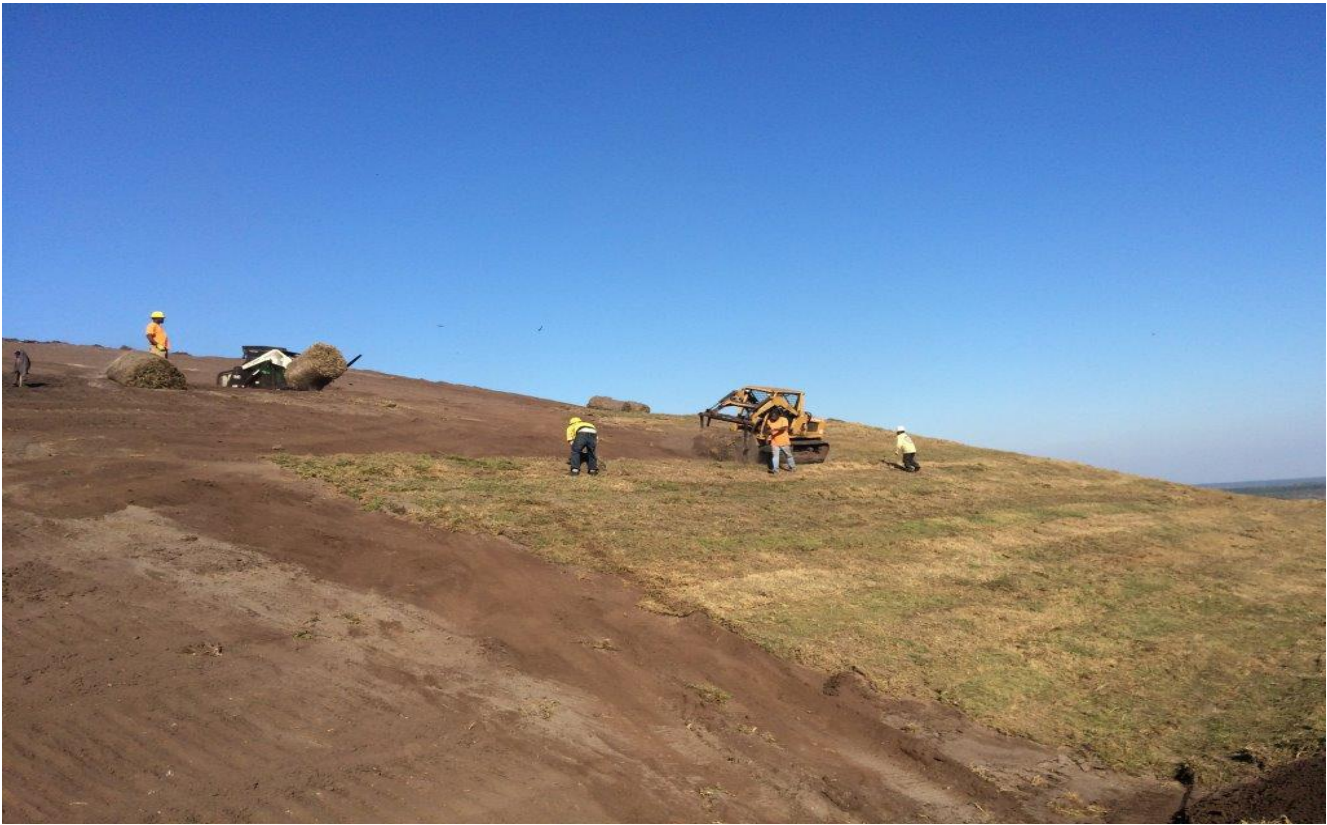
Sodding Unit 92 (facing Easterly) (November 2016)
