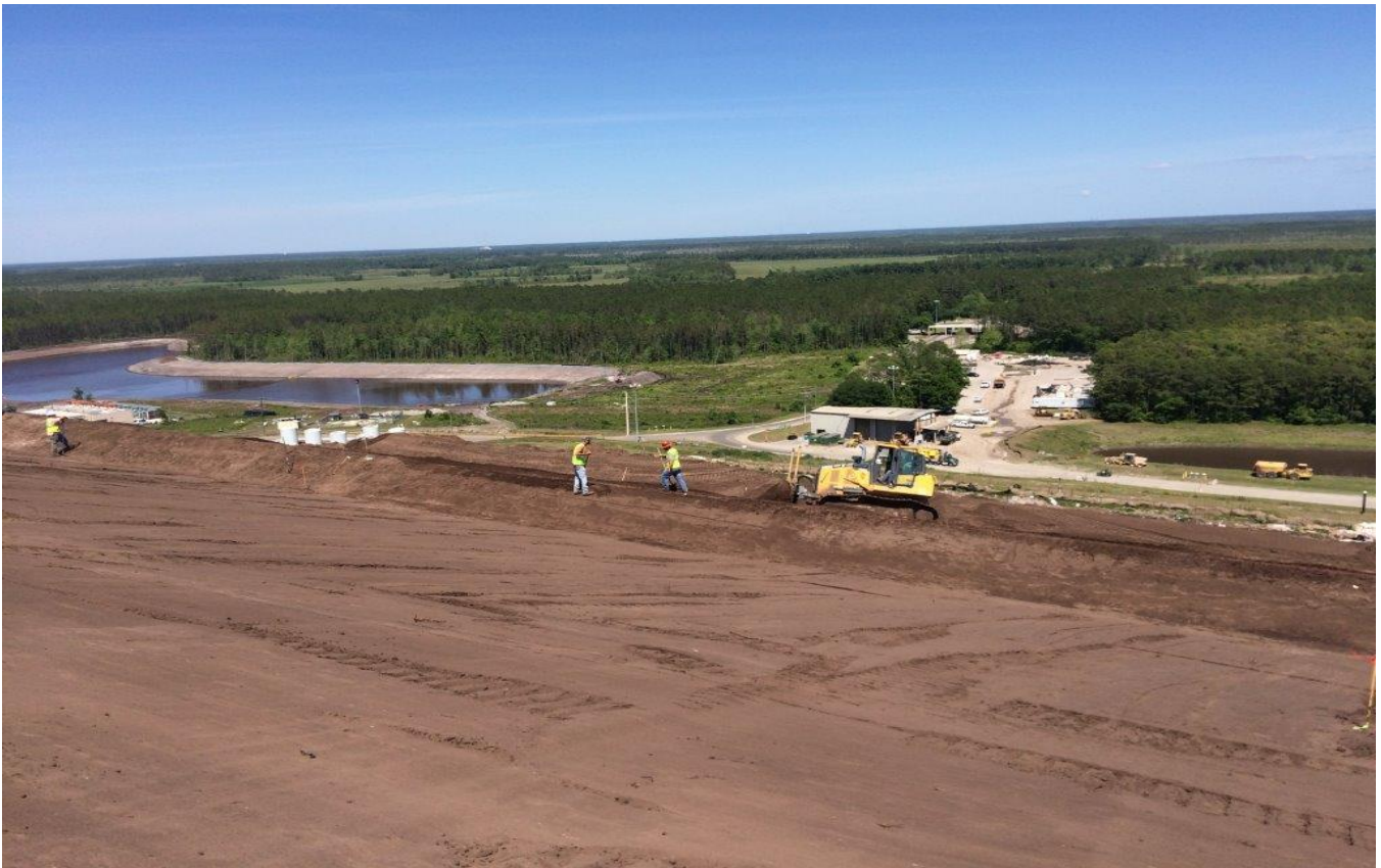
Final Grading Initial Cover – Units 82-84 (Facing Easterly) (April 2016)
