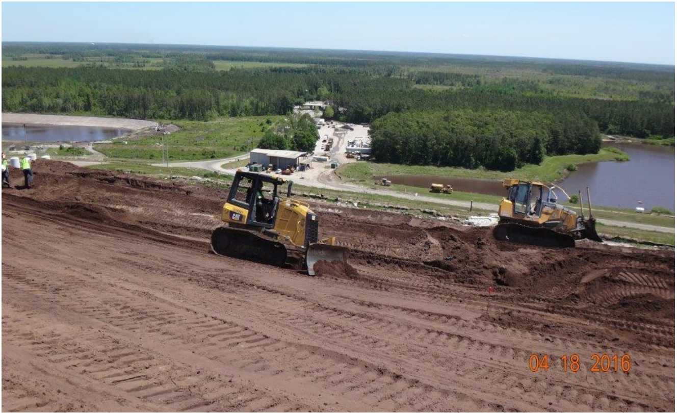
Balancing Initial Cover – Units 82-84 (Facing Easterly) (April 2016)
