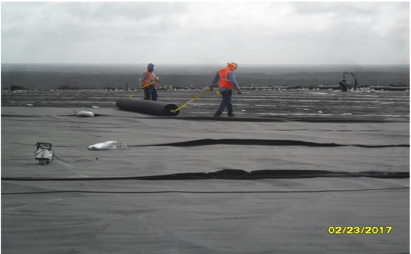
Deployment of geotextile at top of hill (facing Southeasterly) (February 2017)
