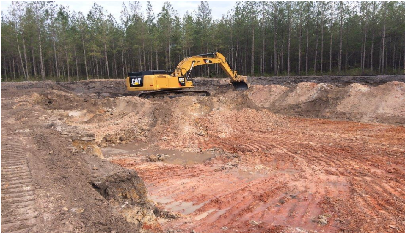
Clay excavation at the Rayonier Borrow Site (NW 257 Street) (April 2016)
