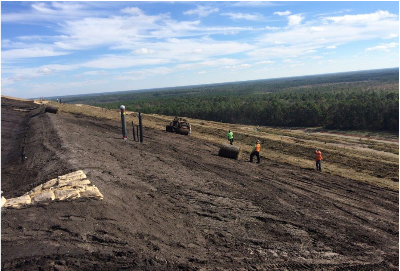
Sod installation Unit 98 (facing Northerly) (December 2016)
