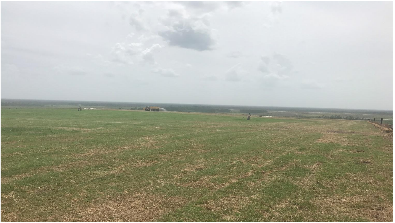
Sod placement – watering truck top of hill (facing Easterly) (May 2017)
