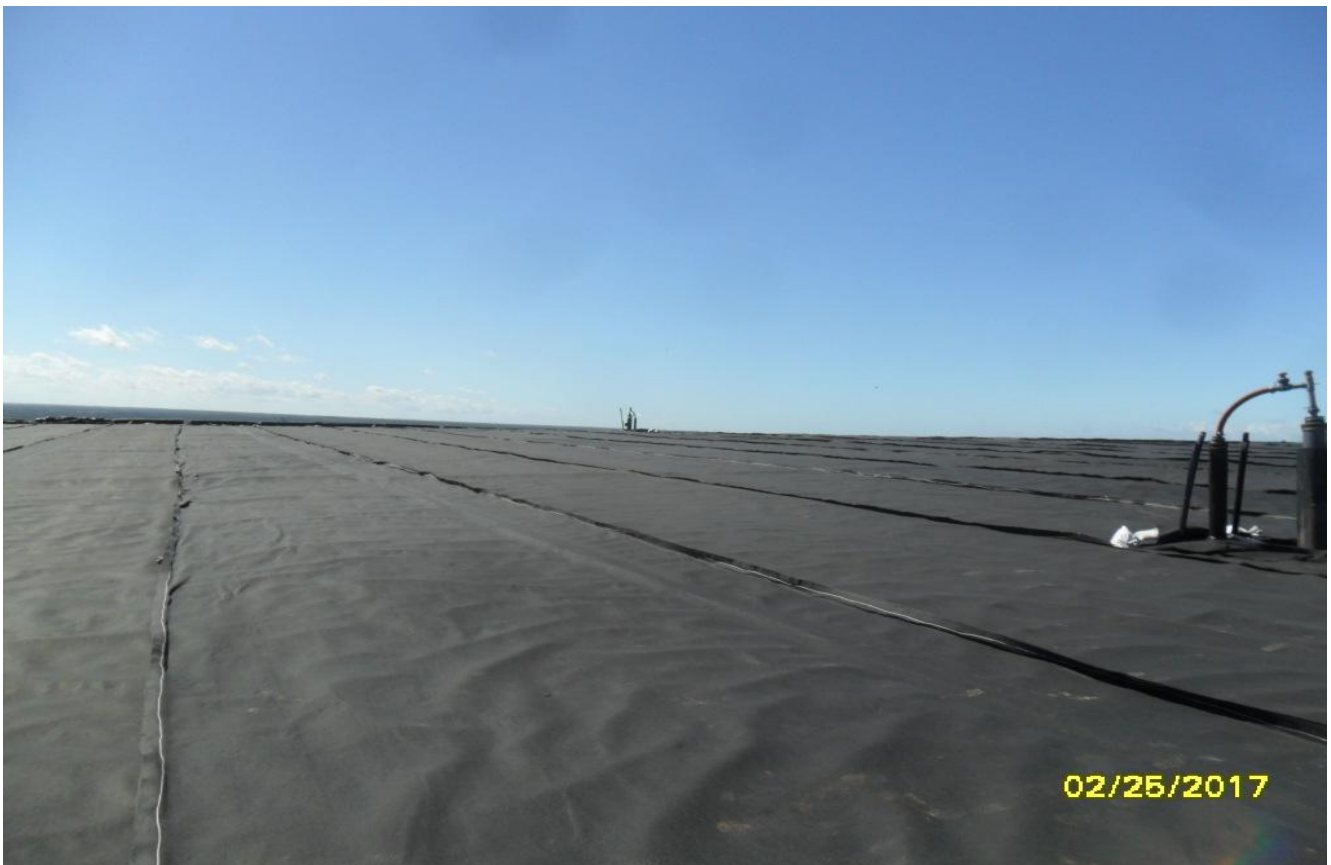
Deployment of geomembrane at top of hill (facing Southerly) (February 2017)
