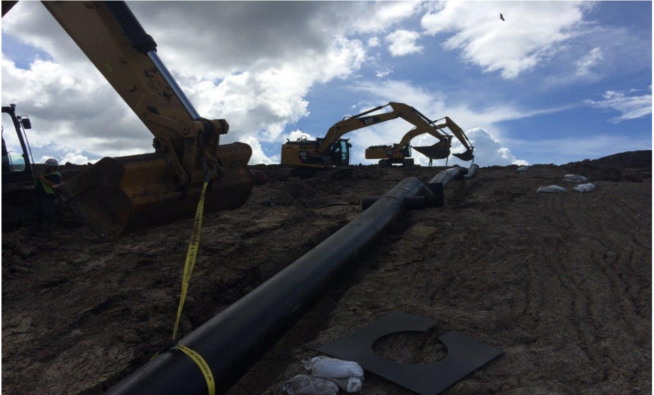
Placing Downcomer D-24 (facing Westerly) (September 2016)
