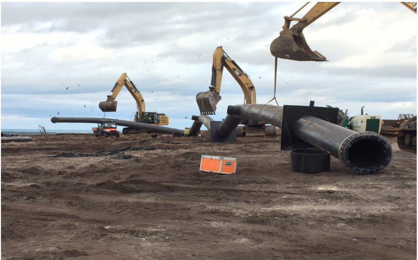
Assembling Downcomer D-52 top of the hill (facing Easterly) (December 2016)
