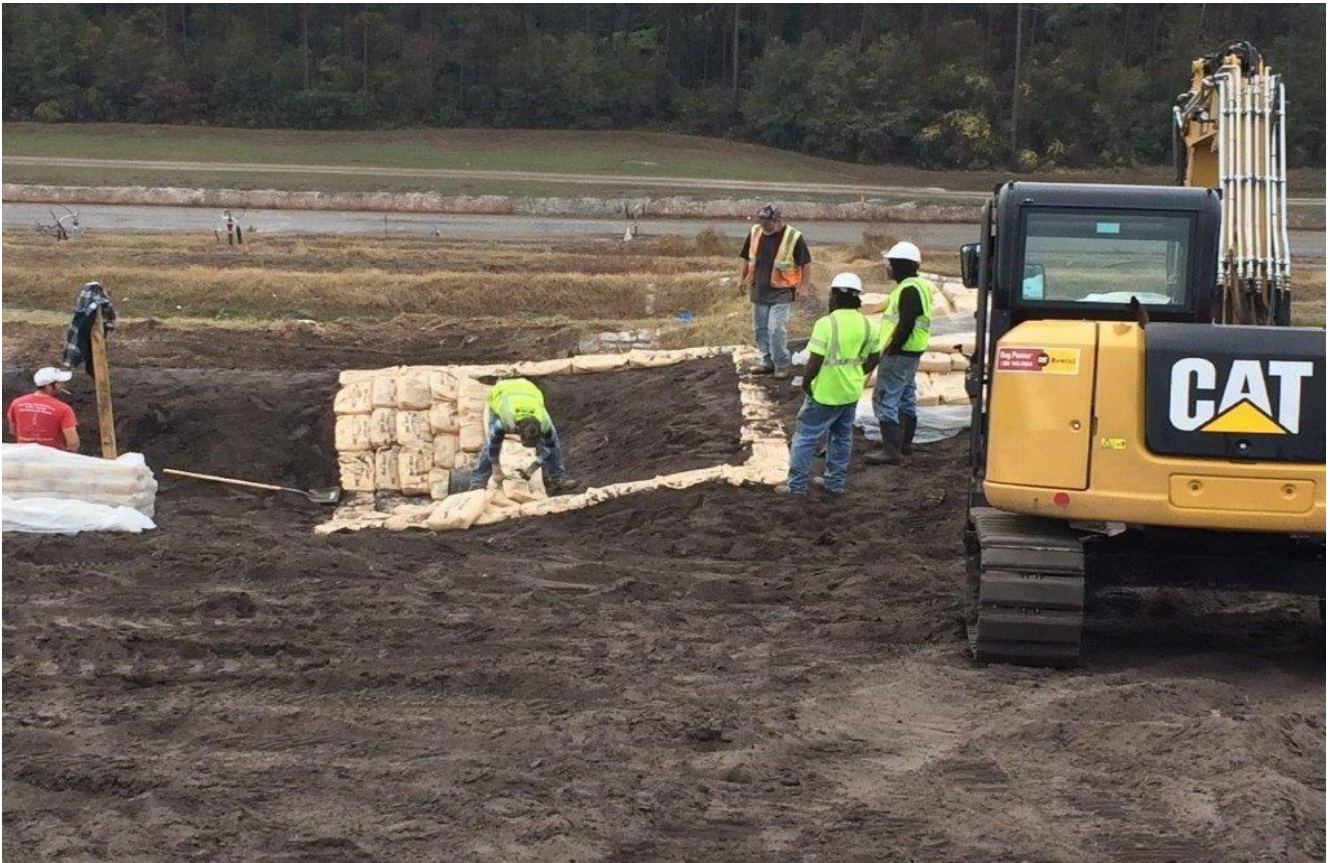
Rip Rap construction at Terrace 8 for Downcomer D-44 (facing Southerly) (December 2016)
