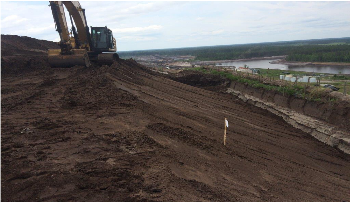
Exposing Clay Tie-In - Unit 83 (Facing Northeasterly) (May 2016)
