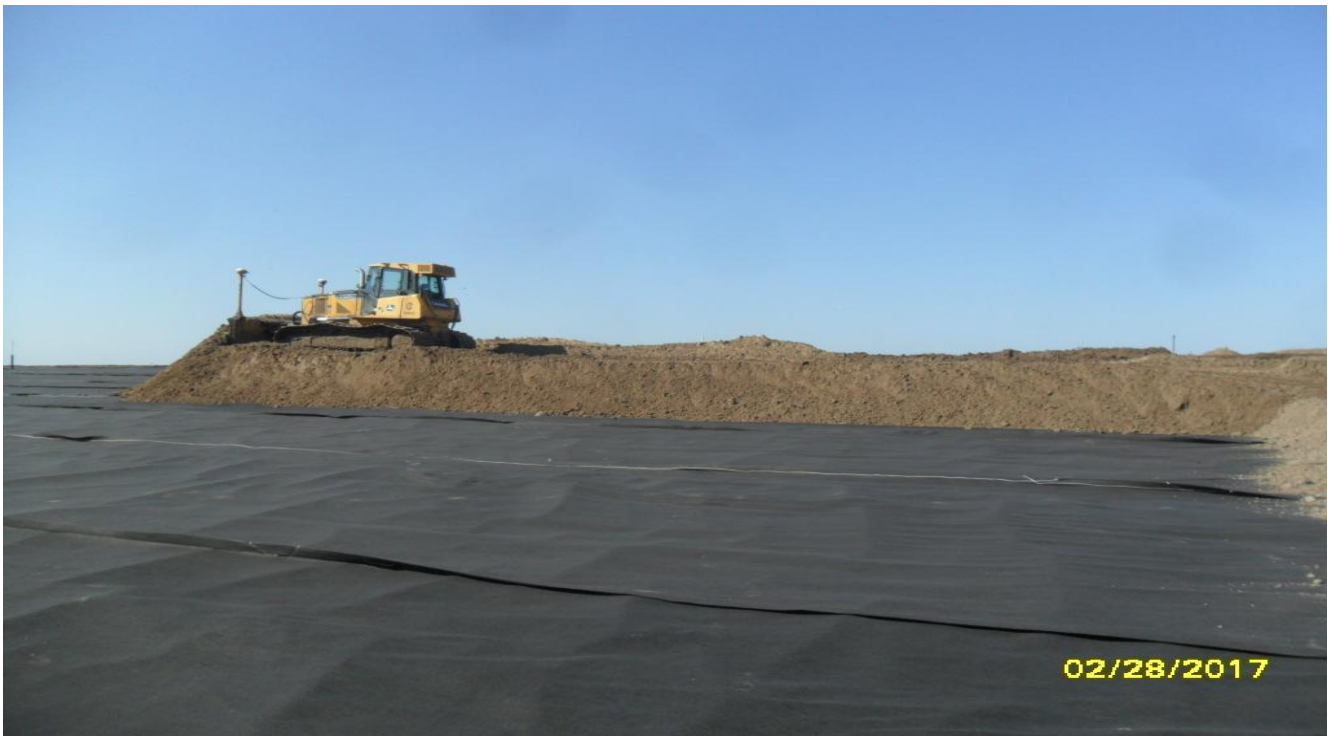
Protective cover placement (facing Northerly) (February 2017)
