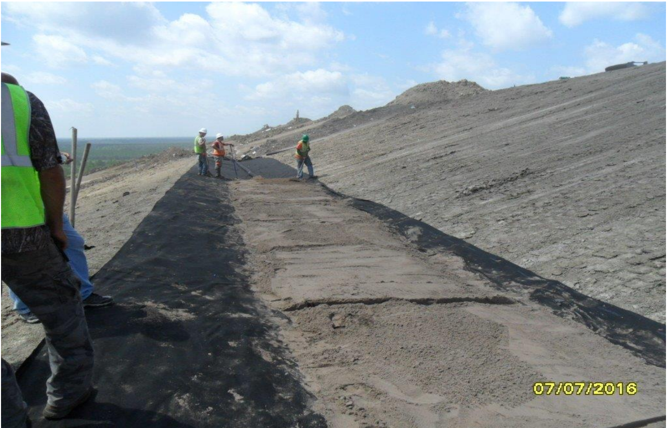
Grading Underdrain sand at Terrace 9 within Unit 84 (Facing Southerly) (July 2016)
