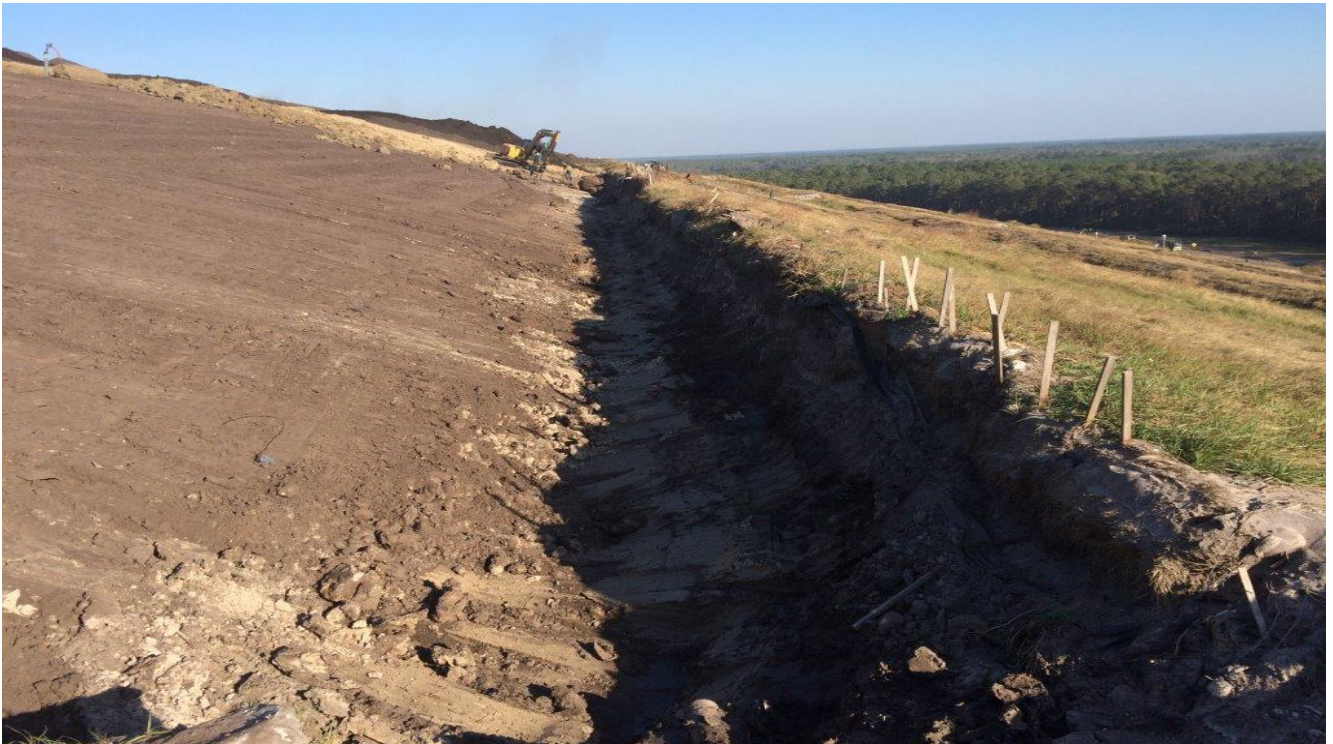
Clay Tie-in at Terrace 7 Unit 100 (facing Easterly) (November 2016)
