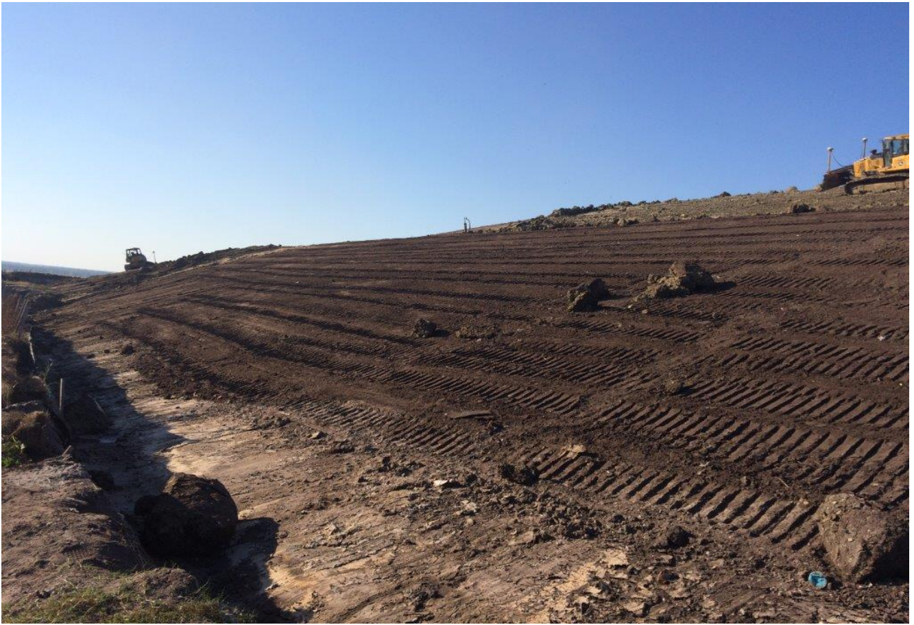
Clay placement Units 97 through 100 (facing Westerly) (November 2016)
