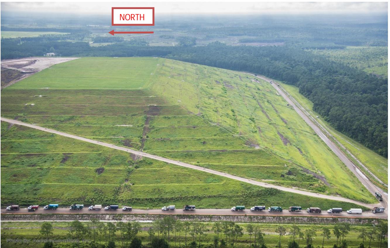
End of Construction - Aerial Photograph - Trail Ridge Landfill (August 2017)
