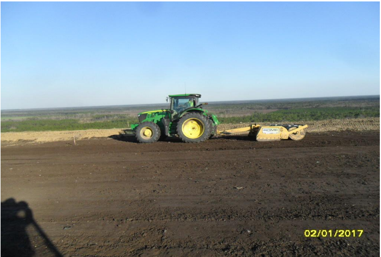
Grading behind Terrace 10 at top of hill (facing Easterly) (February 2017)
