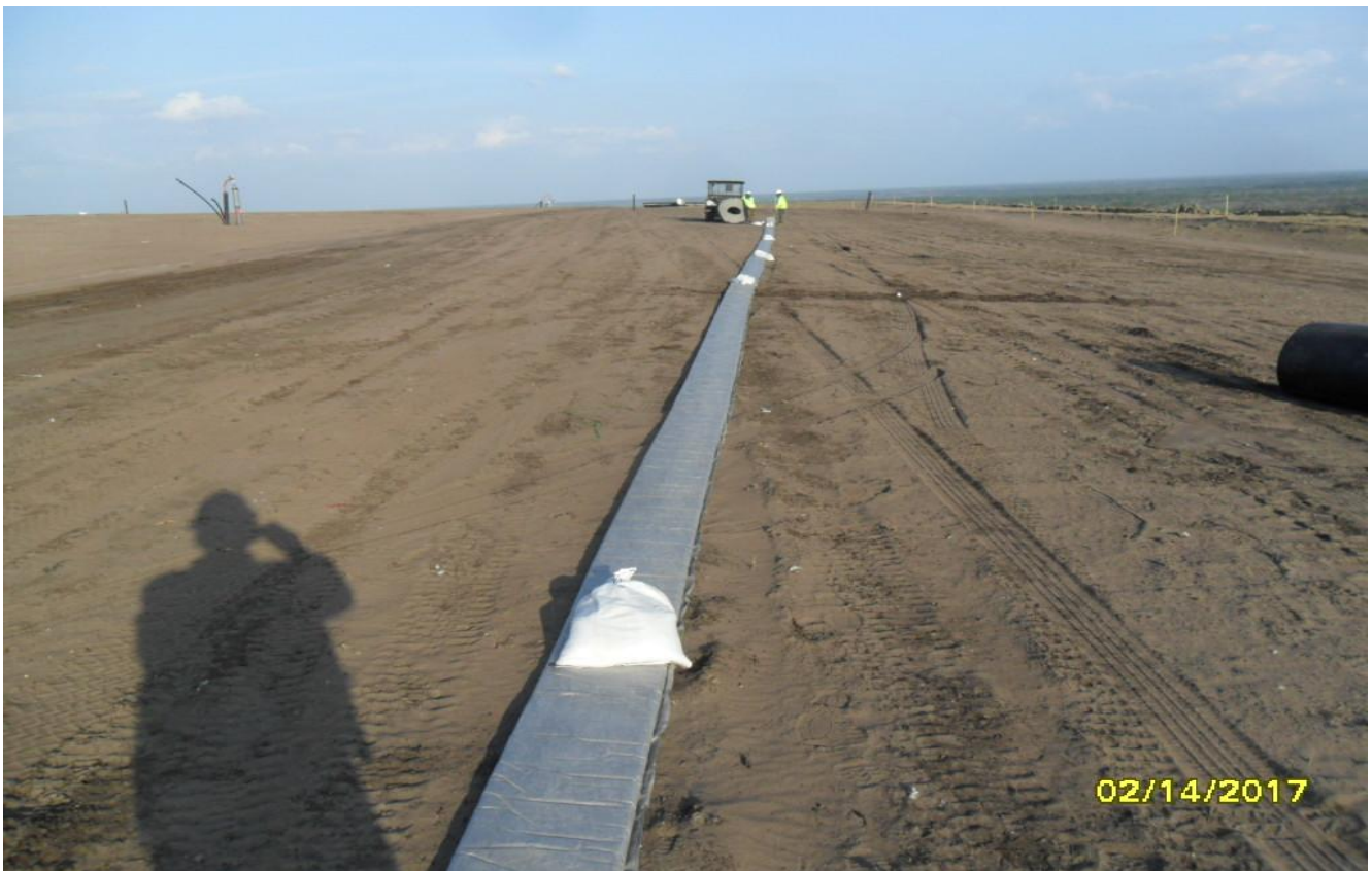
IET installing near surface gas collectors at top of hill (east side) (facing Easterly) (February 2017)
