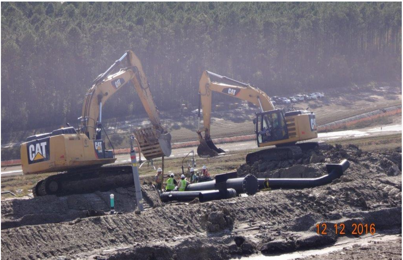
Installation of Downcomer D-47 (facing Southerly) (December 2016)
