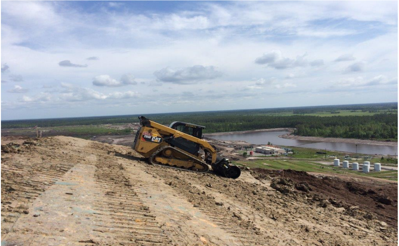
Compacting Clay Test Strip (Facing Southerly) (April 2016)
