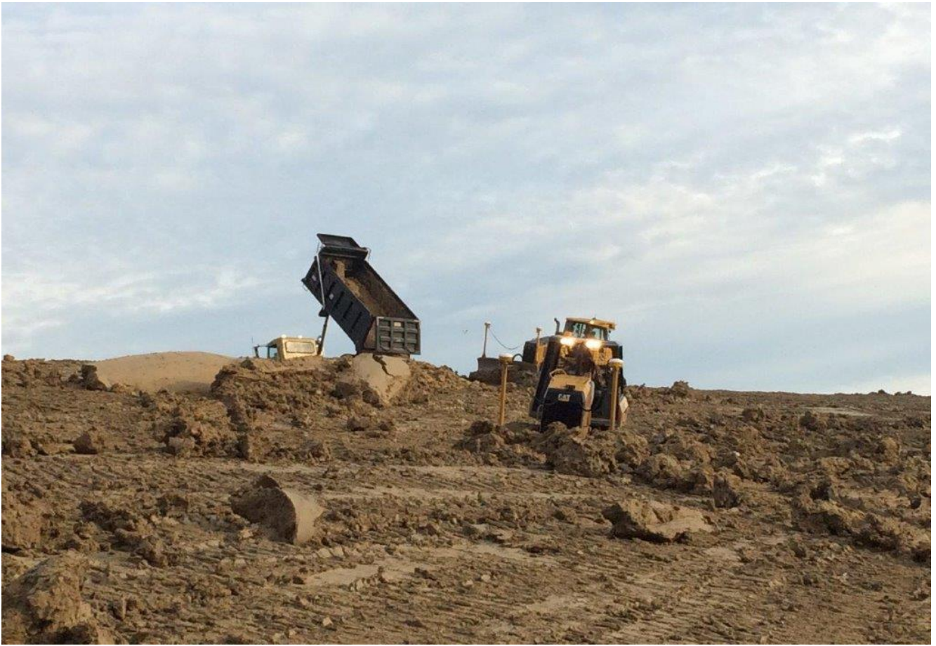
Importing clay Units 106 – 108 (facing Southerly) (December 2016)
