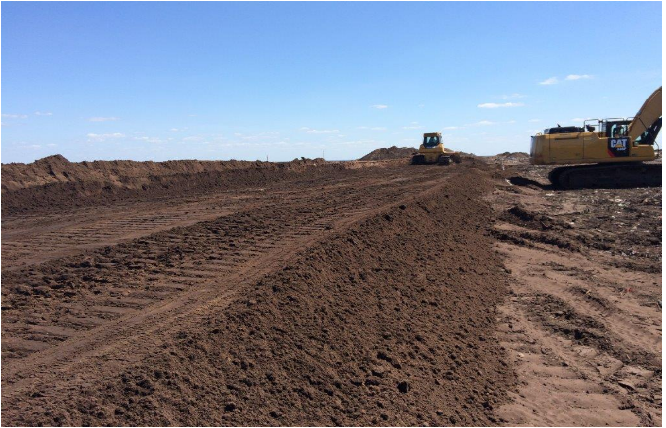
Grading Initial Cover Top Area near Terrace 10 – Units 82-84 (Facing Northerly) (April 2016)
