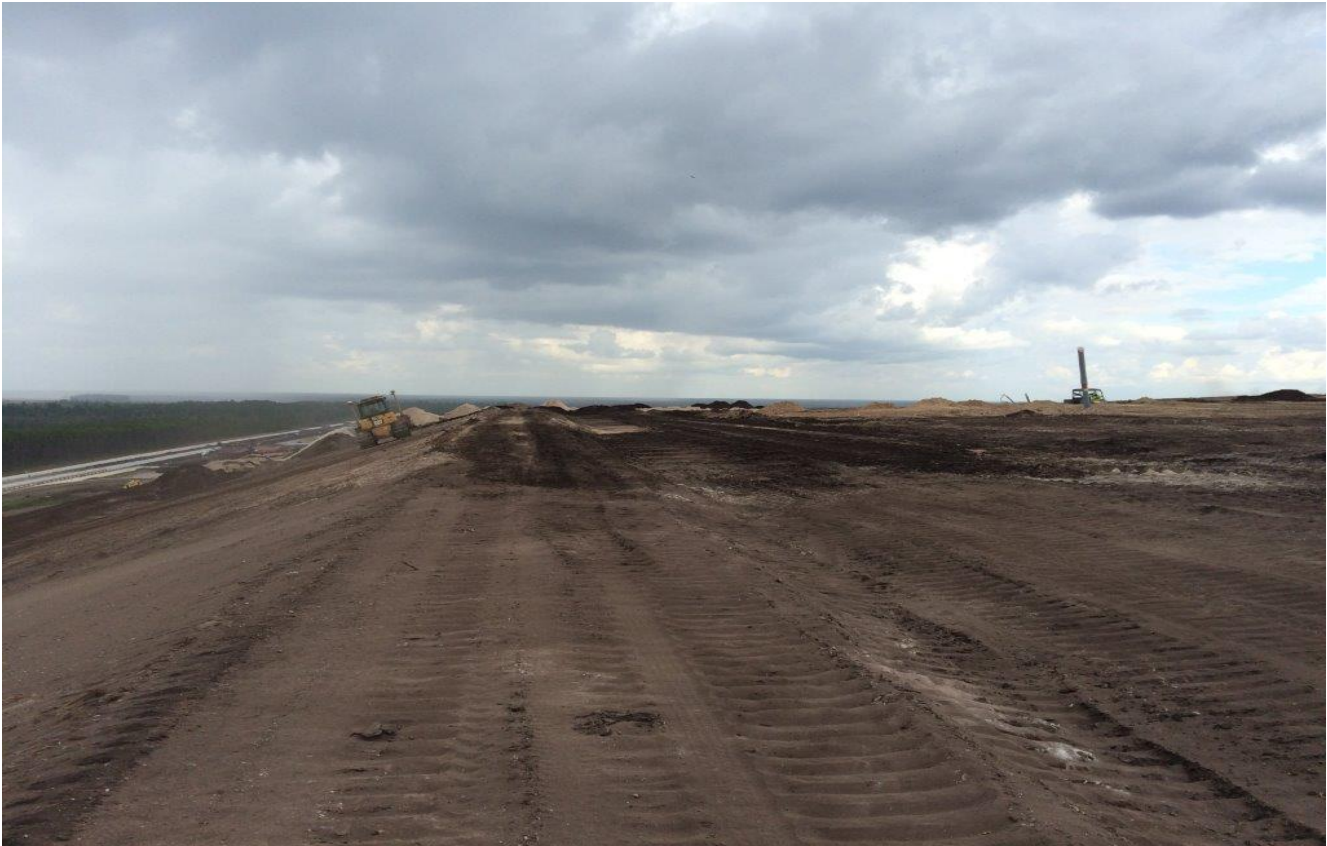
TRLI grading initial cover Unit 108 (facing Northerly) (November 2016)
