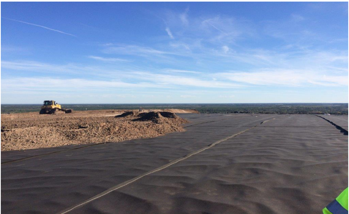
Placement of protective cover top of hill (facing Southerly) (March 2017)
