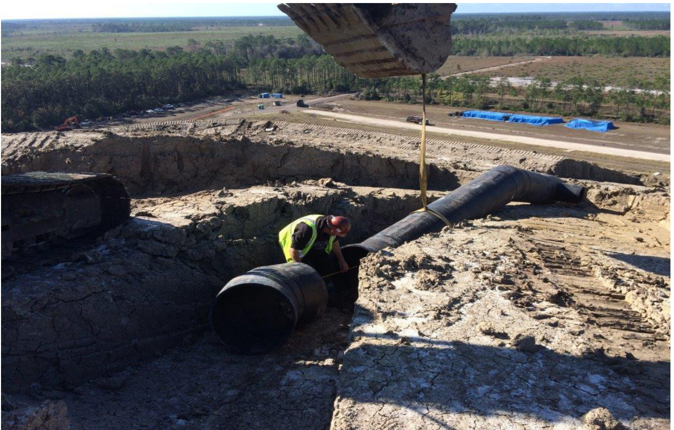
Measuring bend at Downcomer D-52 at Terrace 9 (facing Easterly) (December 2016)
