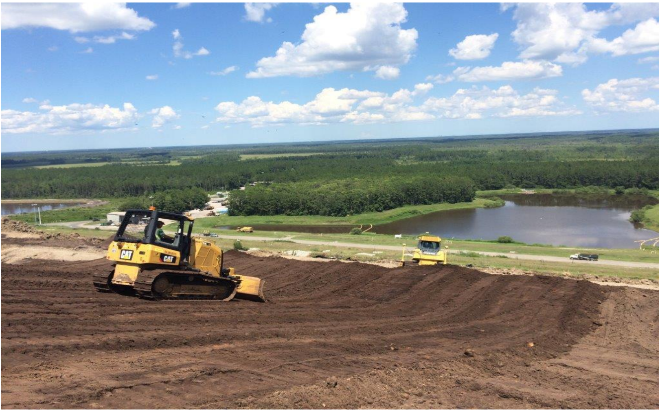
Placement of top soil Unit 87 (Facing Easterly) (July 2016)
