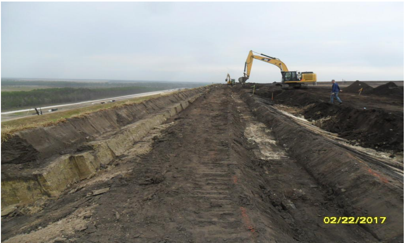
Constructing clay anchor trench at Terrace 10 – Units 105 and 108 (facing Northerly) (February 2017)
