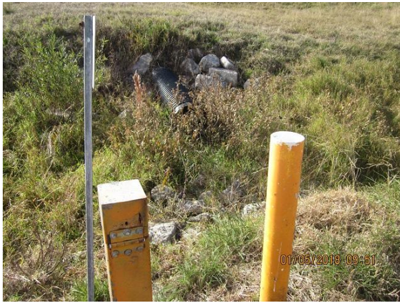
Hazardous Waste Disposal Area
