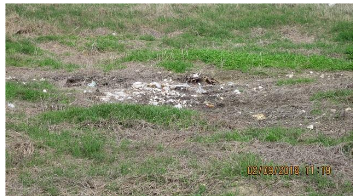
Damaged Cover on Cell 3
