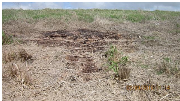
Gas Seepage on Cell 3
