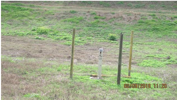
Monitoring Well 11B
