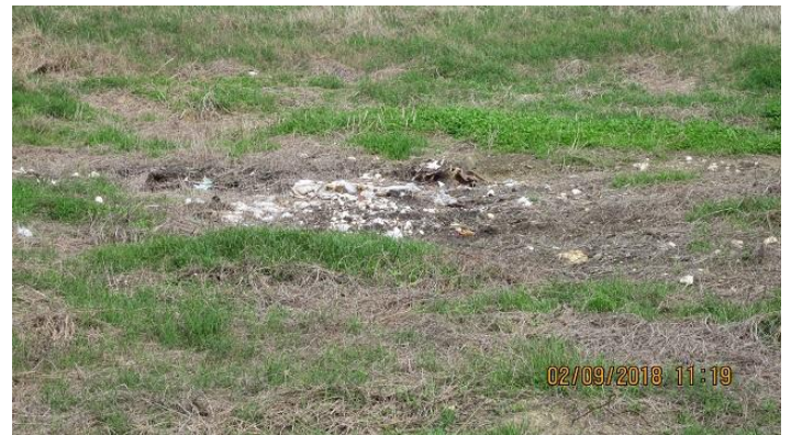
Damaged Cover on Cell 3
