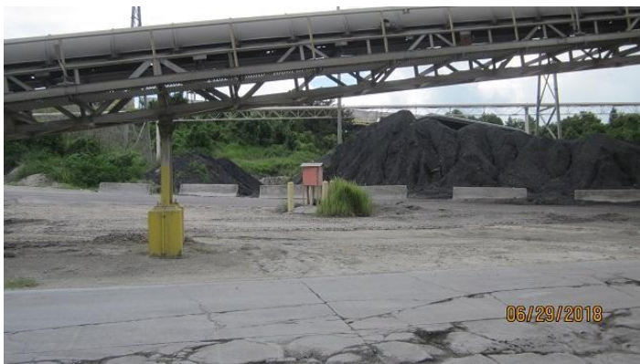
Coal Yard Storage
