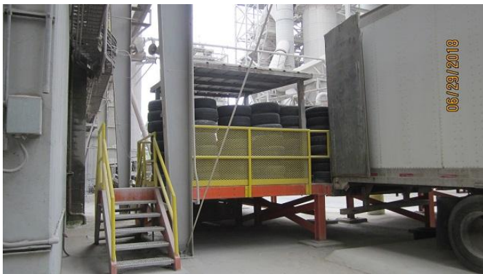
Waste Tire Storage Area - Kiln 1
