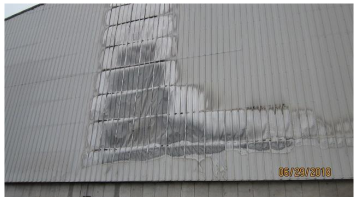
Repaired Fire Damage
