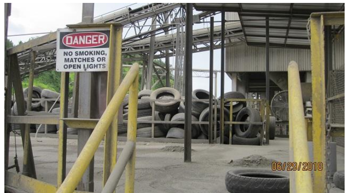
Waste Tire Storage Area - Kiln 2
