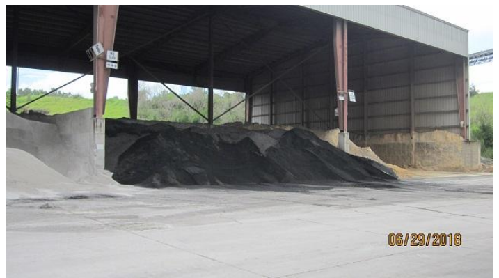
ASB Storage Area
