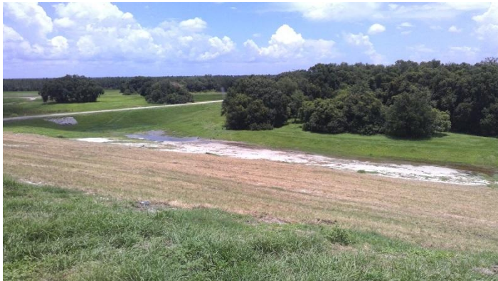
Newly Laid Sod Phase III
