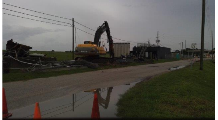
Old Treatment Plant
