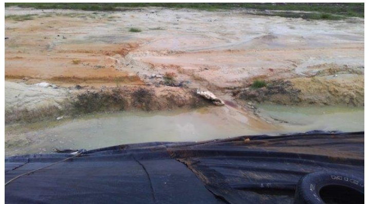
Runoff and Erosion
