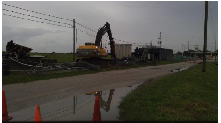
Old Treatment Plant
