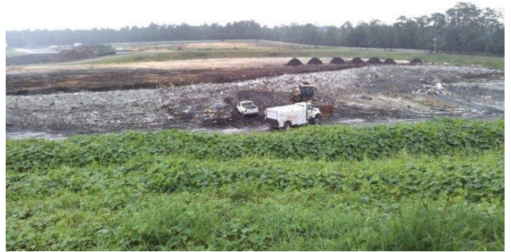
Large Working Face
