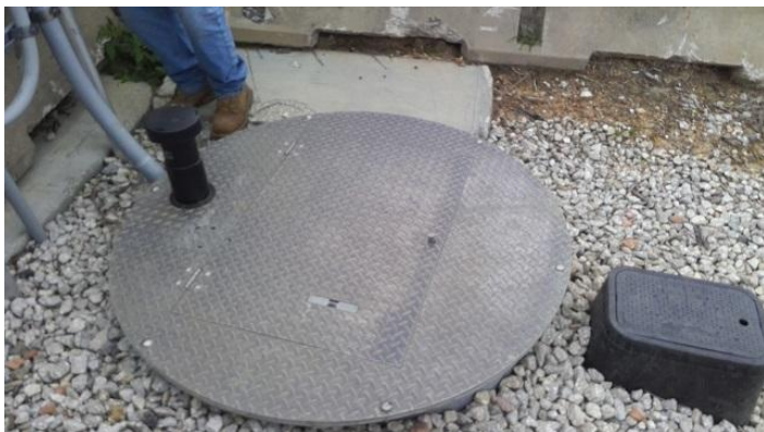
Leachate Toe Drain
