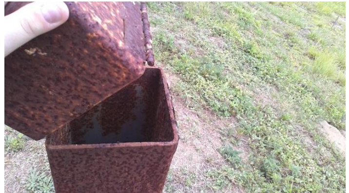
MW-10B: Corroded Hinge
