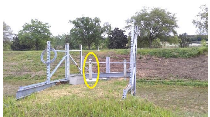
MW-6: Deficient Well Casing
