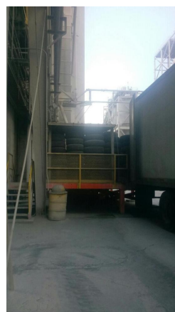
Waste Tire Storage Area - Kiln 1
