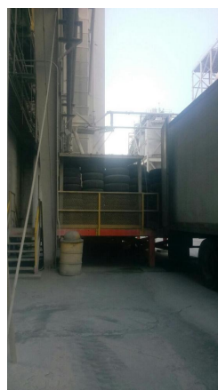
Waste Tire Storage Area - Kiln 1
