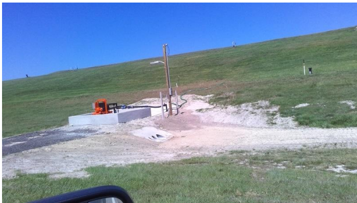
Permanent PS-2 Under Construction
