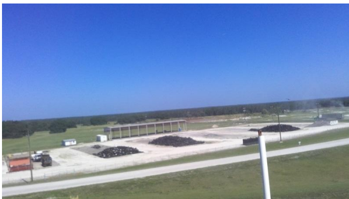
Existing Waste Tire Facility Pad
