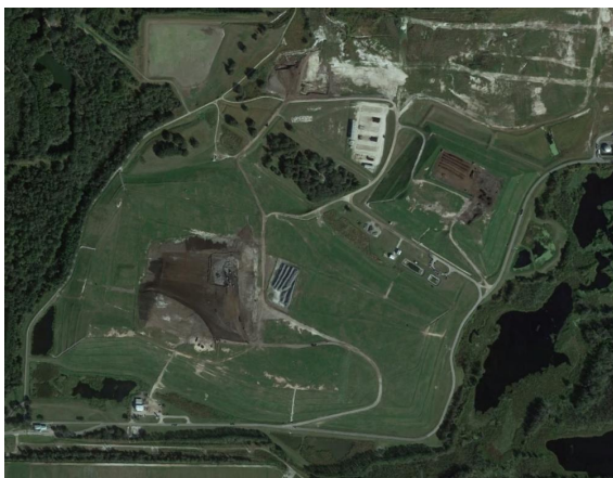
Pump Stations PS-B And PS-A
