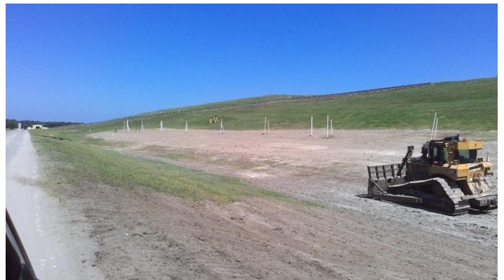
Leachate Cut-off Trench Extension
