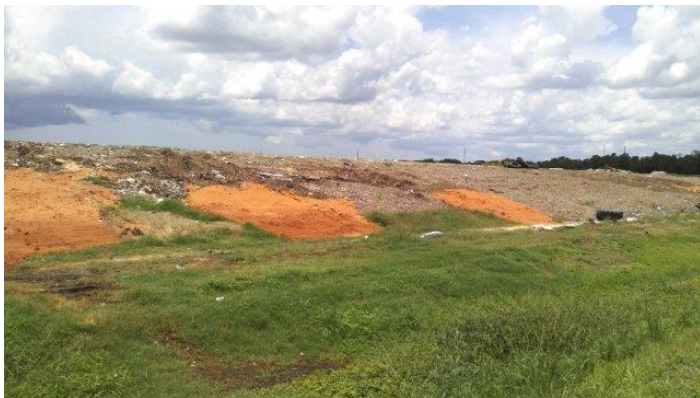
East-Facing Slope Seep
