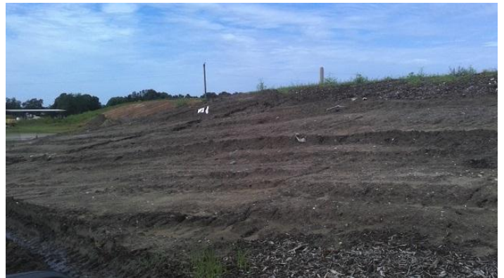
Active Face of Class I Landfill
