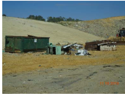
Removing metals for select waste
