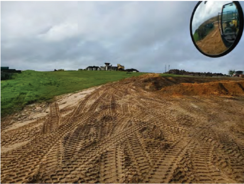
40' Gap Tire Berm
