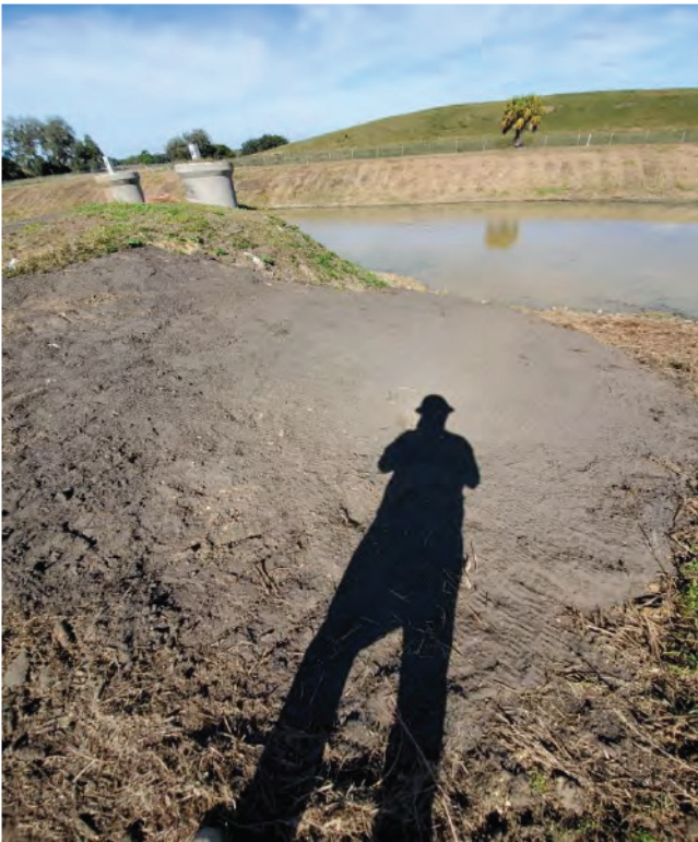
Right (east) side of MW 4 and 4b
