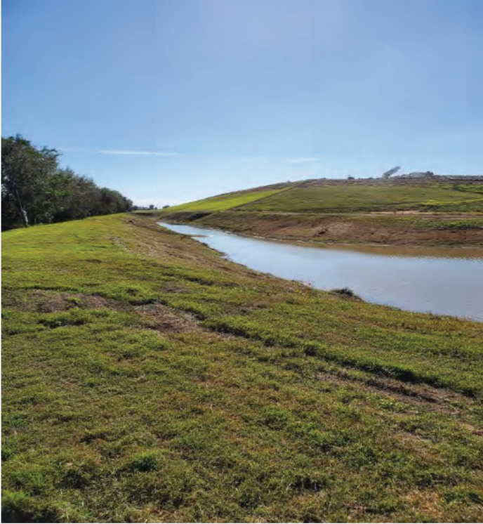
Pond 3 East Side Vegetation Removal and Mowing
