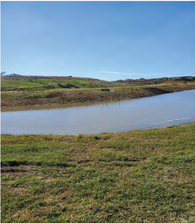
Pond 3 North Side Vegetation Removal and Mowing
