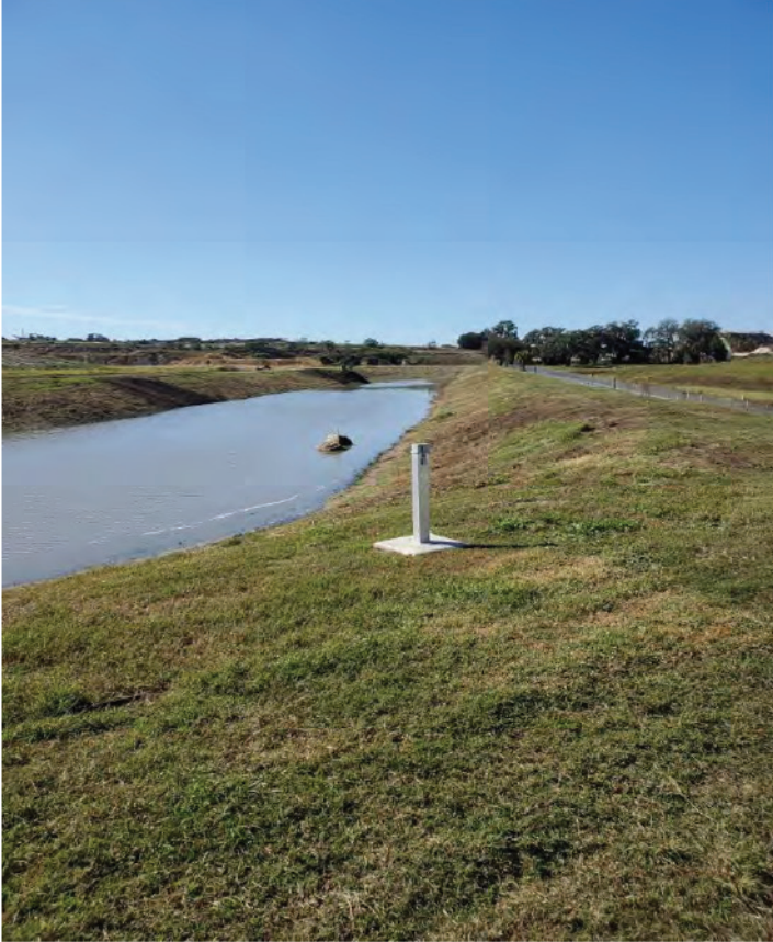
Pond 3 North Side Vegetation Removal and Mowing
