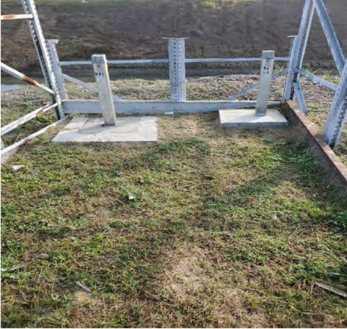
MW6 and 6b Locks
