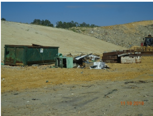
Cell 6-West side slope repair
