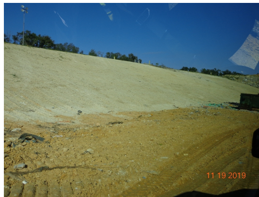
Cell 6 - West side slope repair
