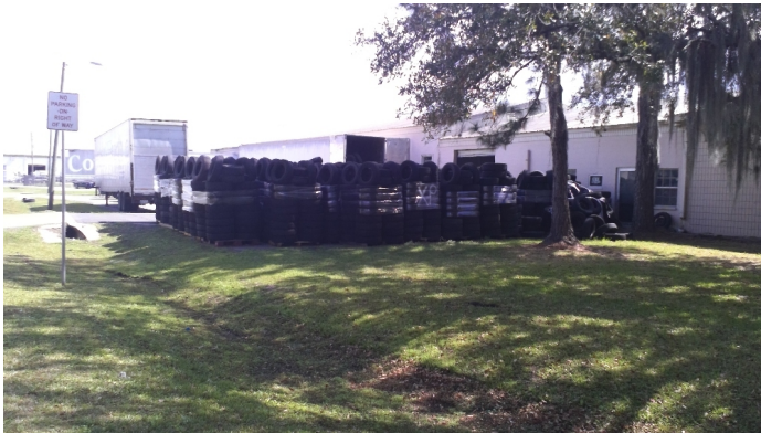
Exterior of S&R Building
