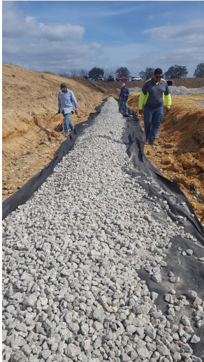
Gravel over pipe prior to wrapping geotextile
