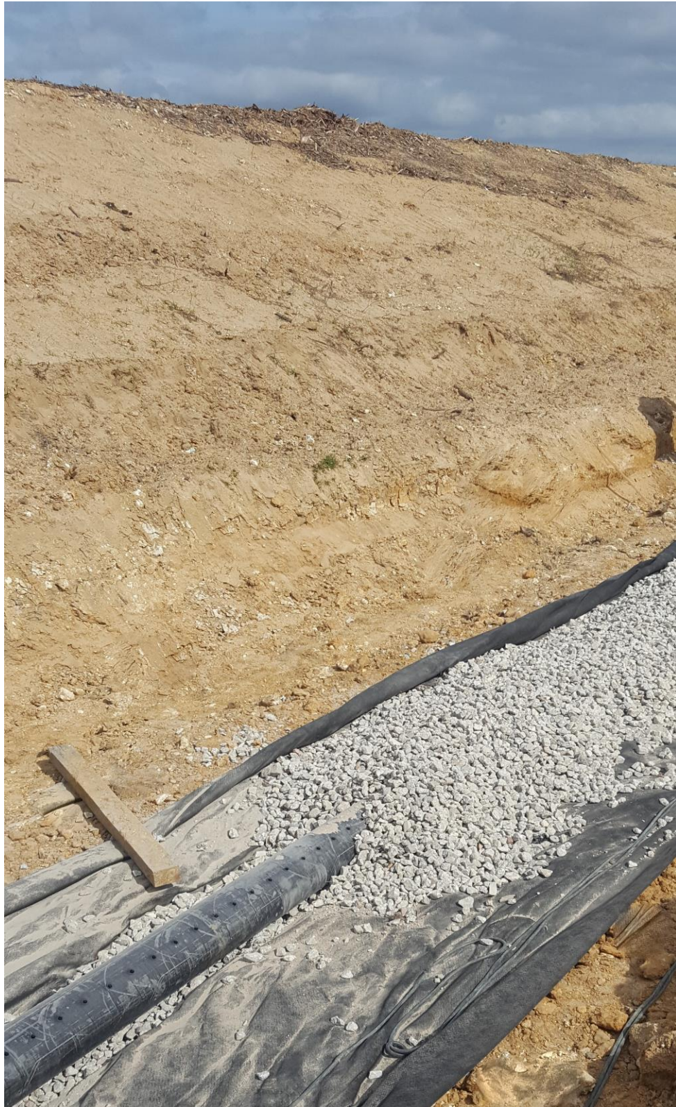
Gravel over pipe prior to wrapping geotextile
