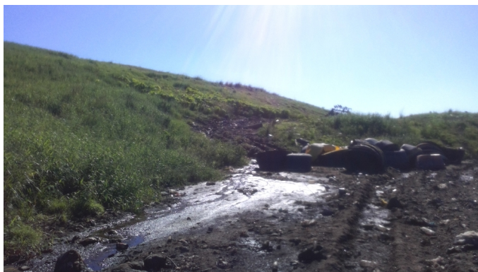
D) Tire Ruts, Ponding
