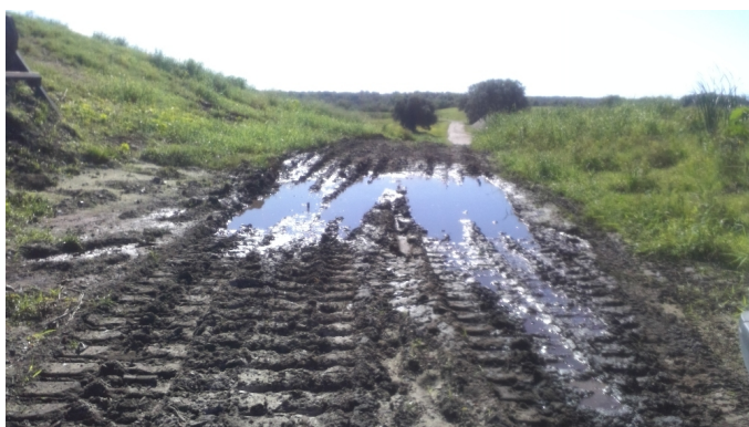
D) Tire Ruts, Ponding
