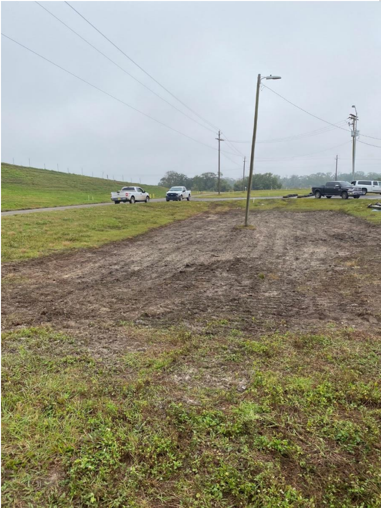
Photo 3. Completed clean soil backfill of affected area (Looking NE).
