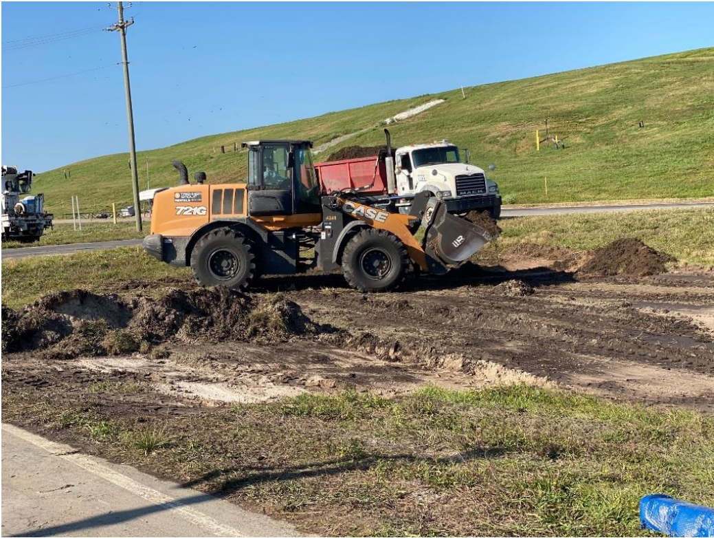
Photo 2. Affected soil removal (Locking NW)
