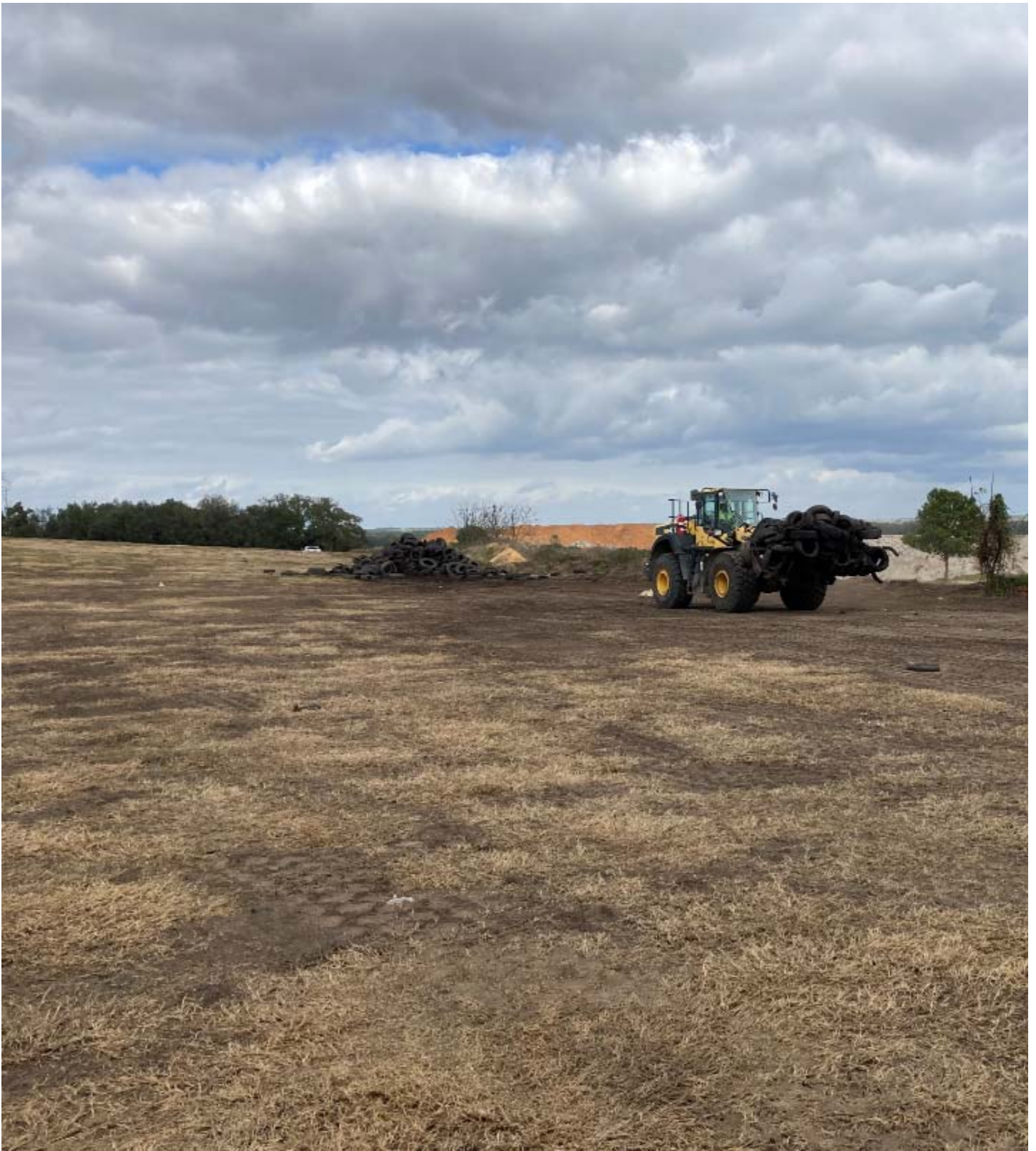
2 Waste tires being removed from temporary stockpile
