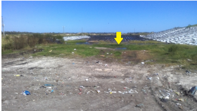
2020 - Collapsed Berm
