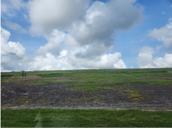
Lack of Cover on E Slope Stage II
