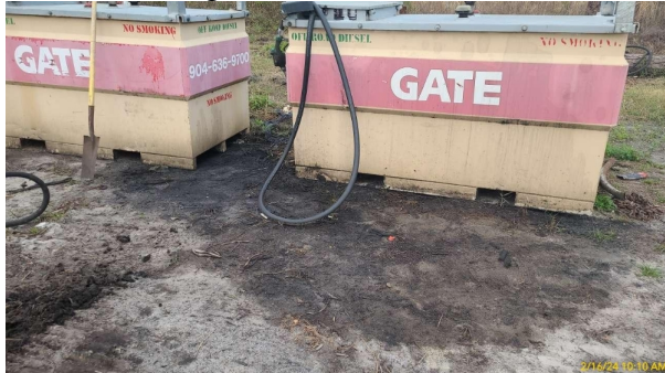
Diesel Staining
