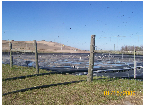
Leachate Ponds at the Site
