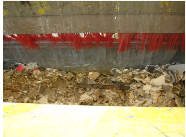
Transfer Station drywall load
