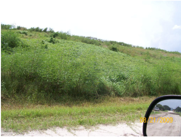
Portion of Eastern Slope
