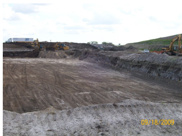
Excavation between Stage I & III
