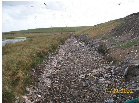
bermed area (toe of E. side slope)
