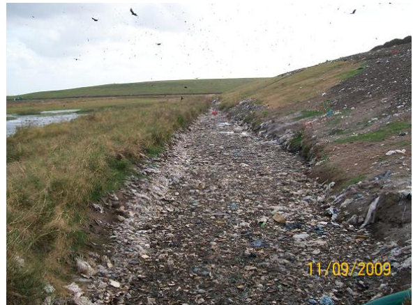
bermed area (toe of E. side slope)
