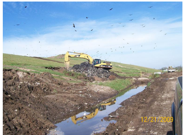
Leachate Seeps Being Repaired
