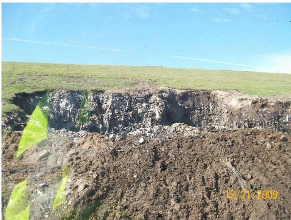
Leachate Seeps Being Repaired
