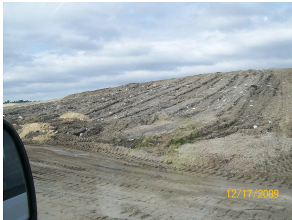
Inadequate initial cover.
