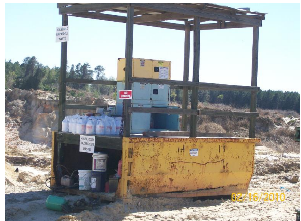
Unacceptable Waste Storage
