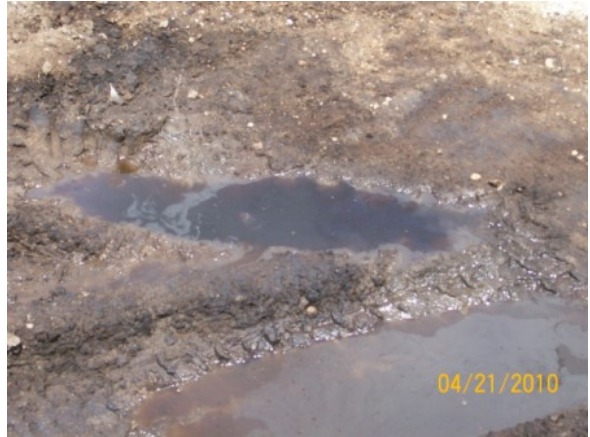
Leachate seep at toe of slope
