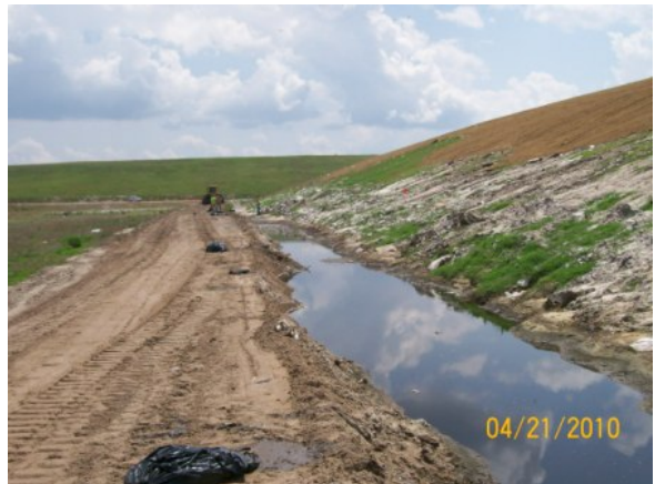
E side slope ditch and berm
