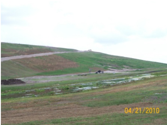
New haul road
