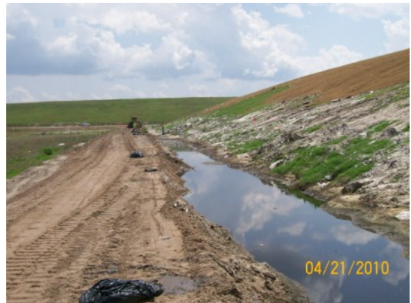
E side slope ditch and berm
