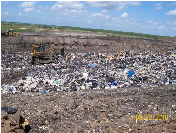
Lower Portion of Working Face
