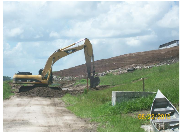
Cell 6 Seepage Repairs
