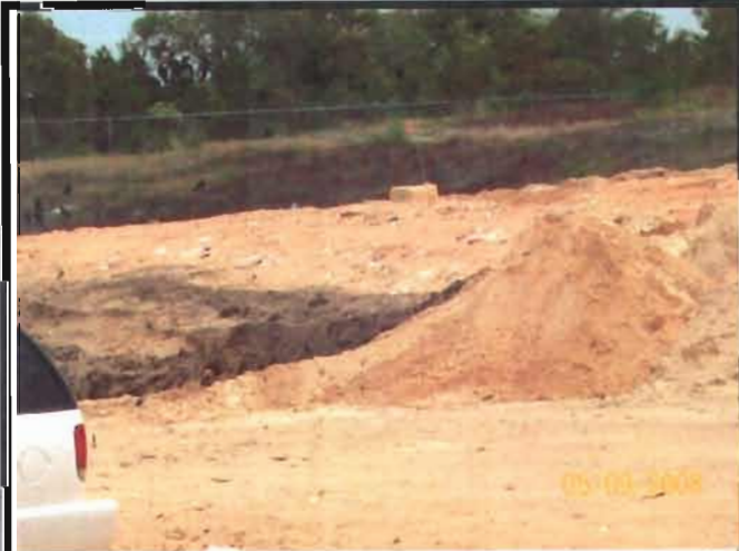
Phase II active area - exposed waste outside of the traffic pattern.
