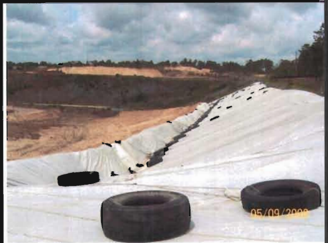
Phase II - working face viewed from atop eastern side.
