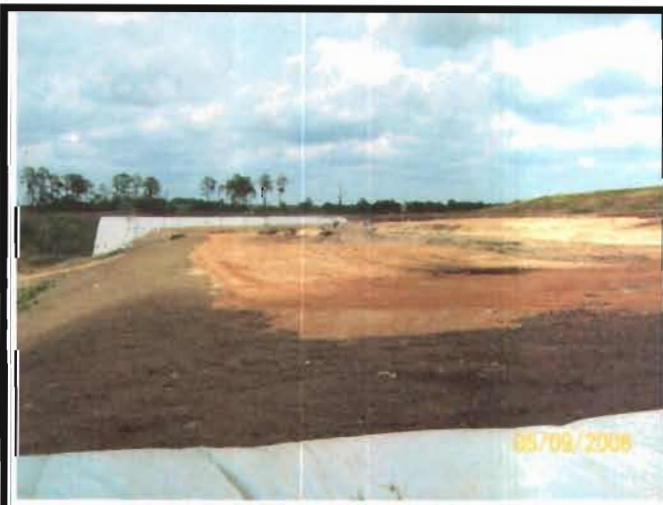
Phase II – viewed from the NW corner
