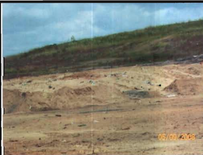
Phase II active area - exposed waste outside of the traffic pattern.
