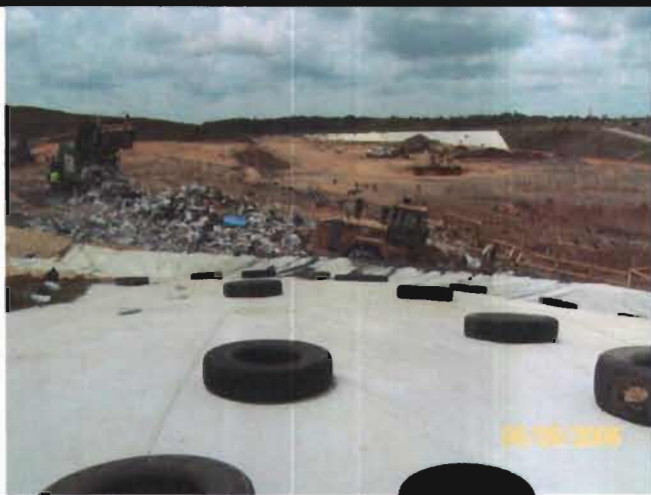
Phase II - working face viewed from atop eastern side.
