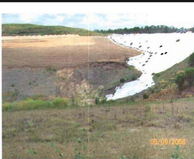
Phase II - viewed from the North.
