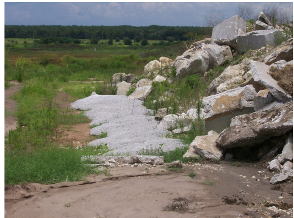
concrete truck washout
