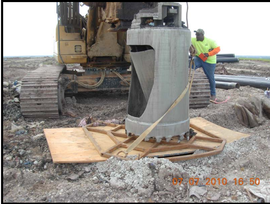
Photograph 11: Covering extraction well GW-45 bore hole.
