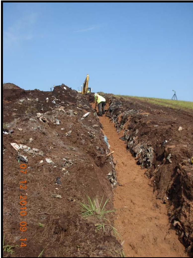
Photograph 35: Applying sand to lateral trench from GW-49 to GW-50.
