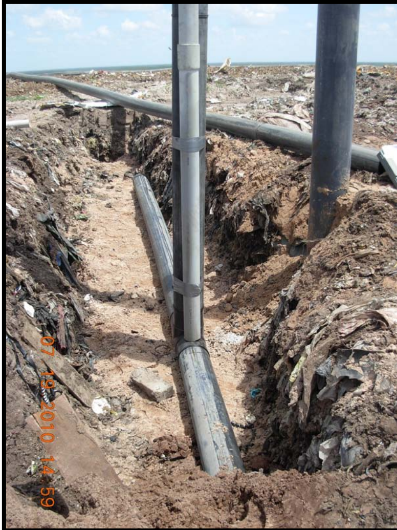
Photograph 45: Lateral riser to GW-21 with tee and 10 foot lateral stub-out for future tie-in.
