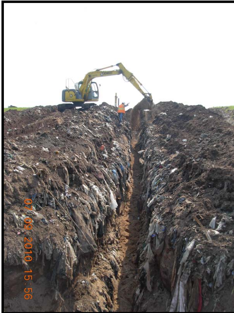
Photograph 28: Sanding trench for lateral to extraction well GW-45.
