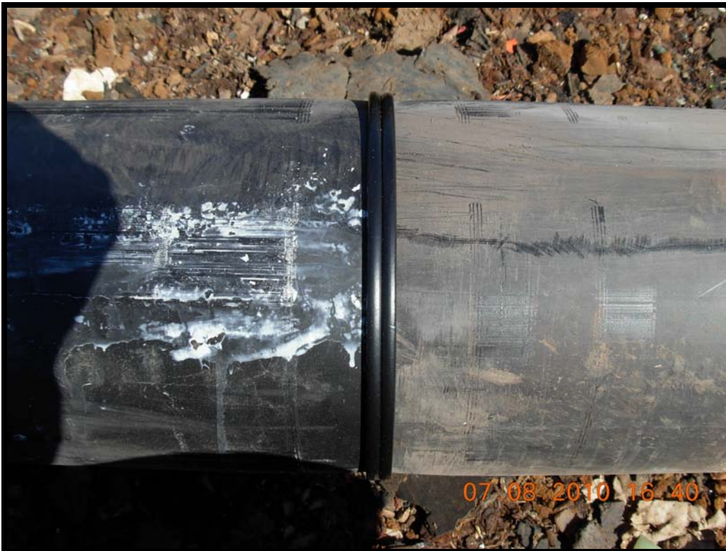
Photograph 14: 6" HDPE SDR 17 lateral hard weld showing acceptable bead.
