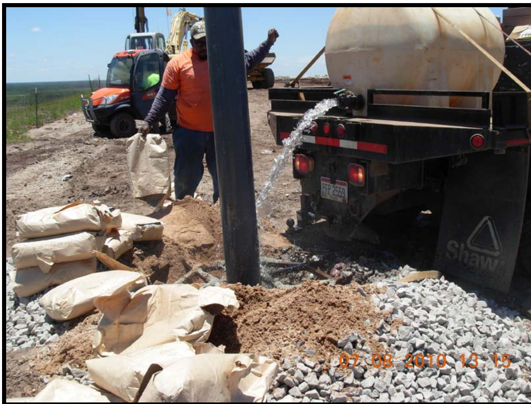
Photograph 22: Hydrating bentonite plug #2 at extraction well GW-45.
