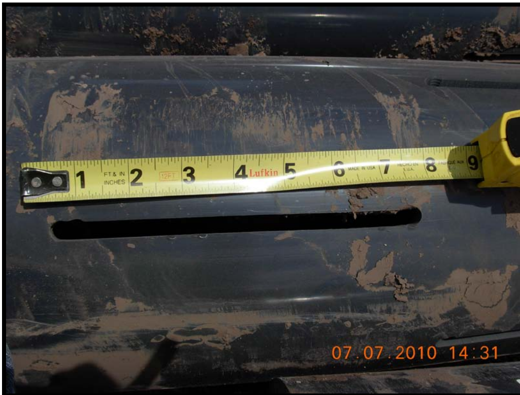
Photograph 6: 8" SCH 80 PVC slot length.
