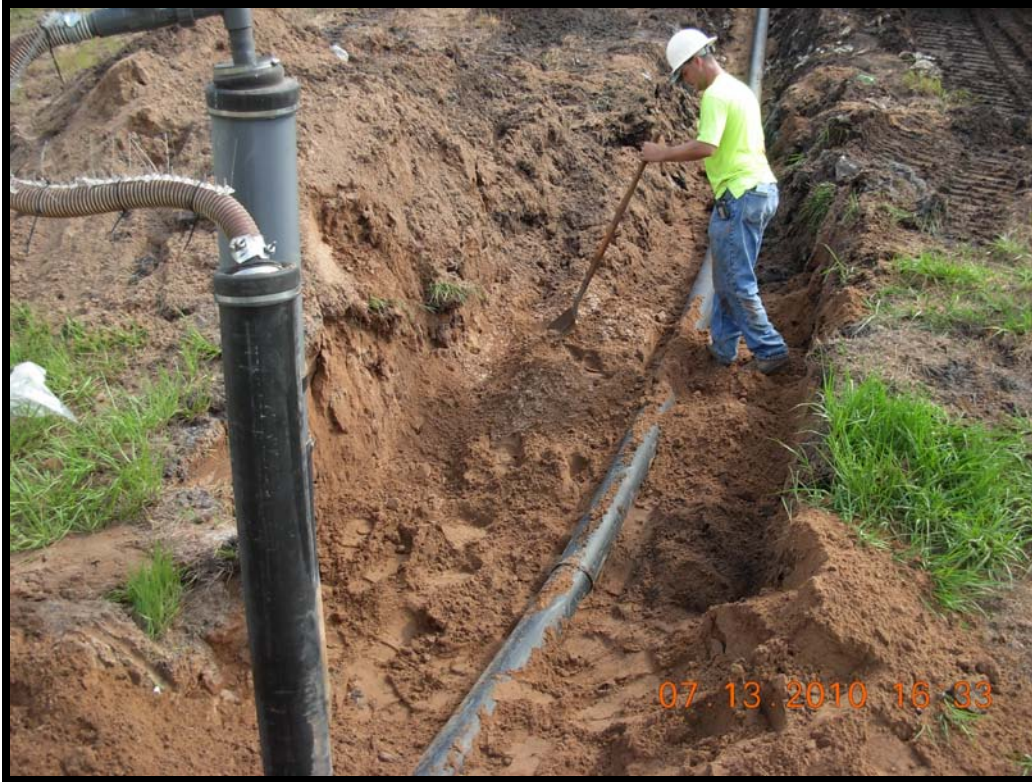
Photograph 36: Sanding trench for lateral from tie-in location at GW-39 to GW-40R.
