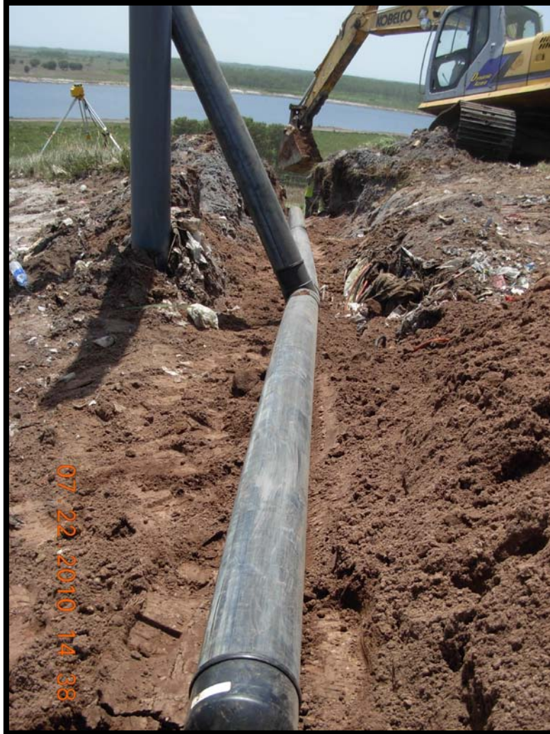
Photograph 59: Lateral riser to GW-35 with tee and 10 foot lateral stub-out for future tie-in.
