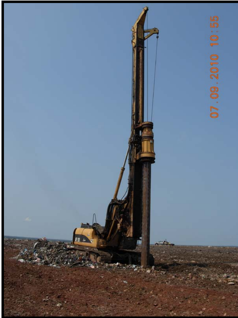
Photograph 27: Drilling extraction well GW-51.
