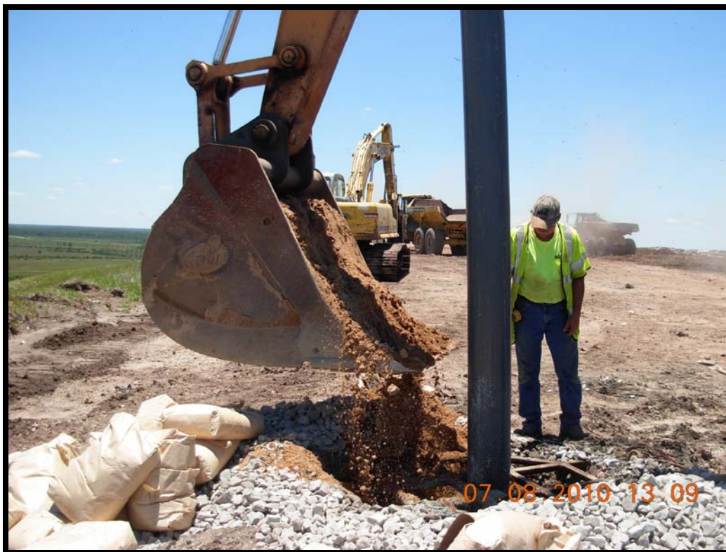
Photograph 20: Adding sandy soil backfill in between bentonite plugs at GW-45.
