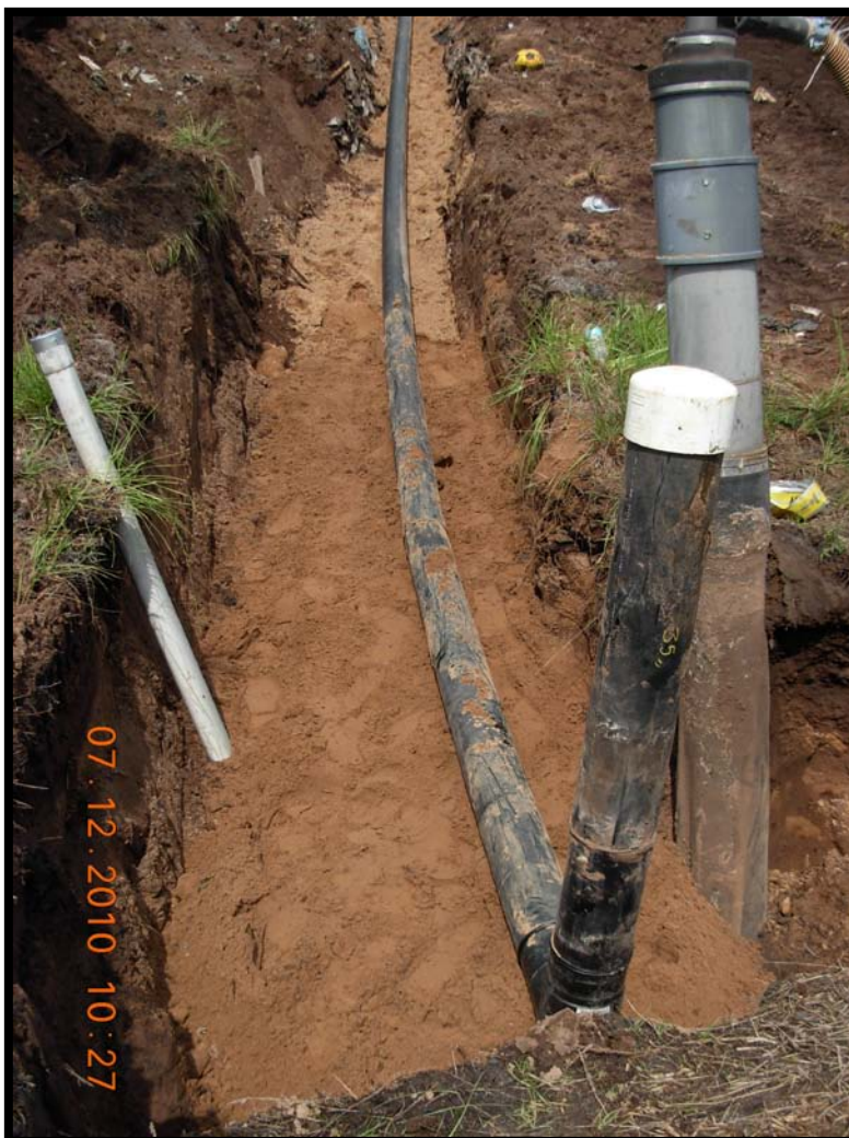
Photograph 33: Tie-in to GW-49 lateral riser for lateral to GW-50.
