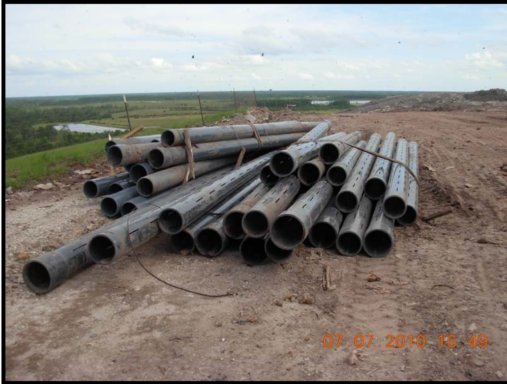
Photograph 3: 8" SCH 80 PVC solid and slotted pipe inventory.
