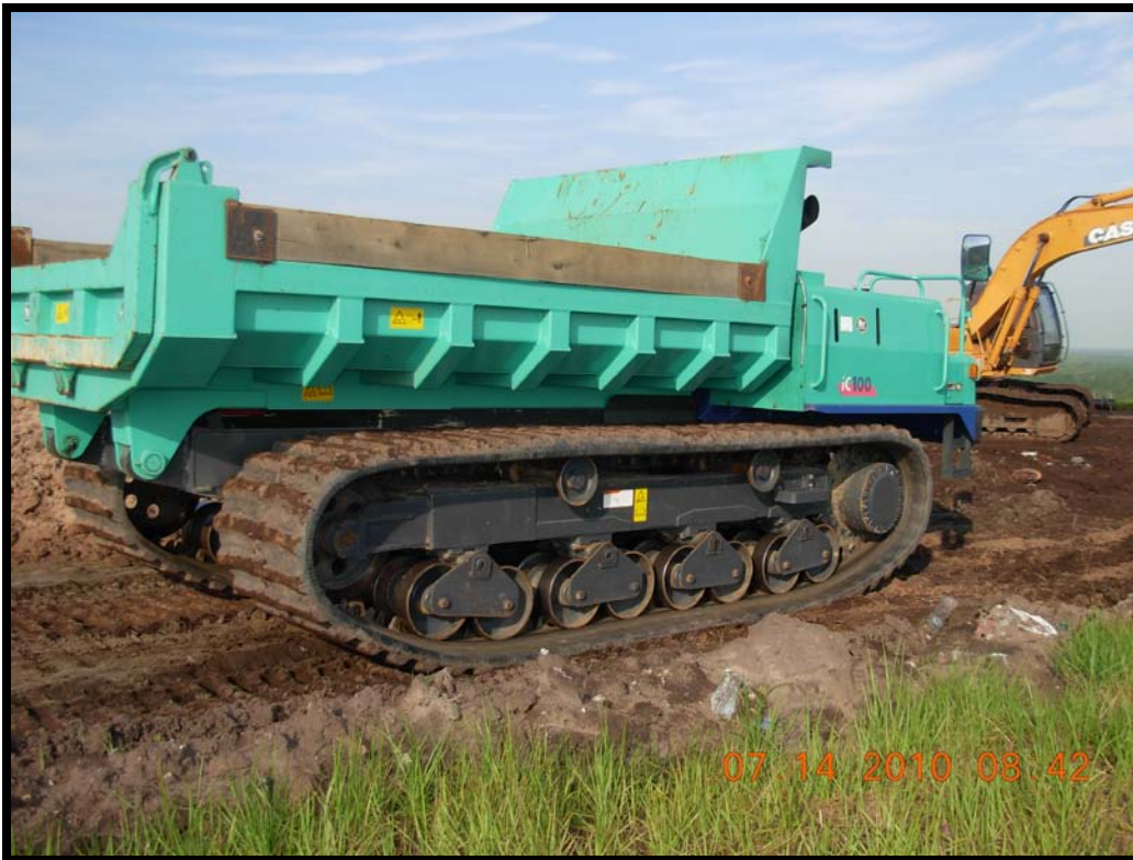
Photograph 37: Track truck ic 100 arrives on site July 14, 2010.
