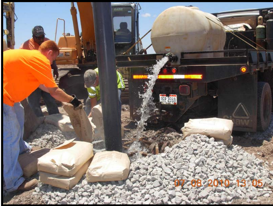
Photograph 19: Hydrating bentonite plug #1 at extraction well GW-45.
