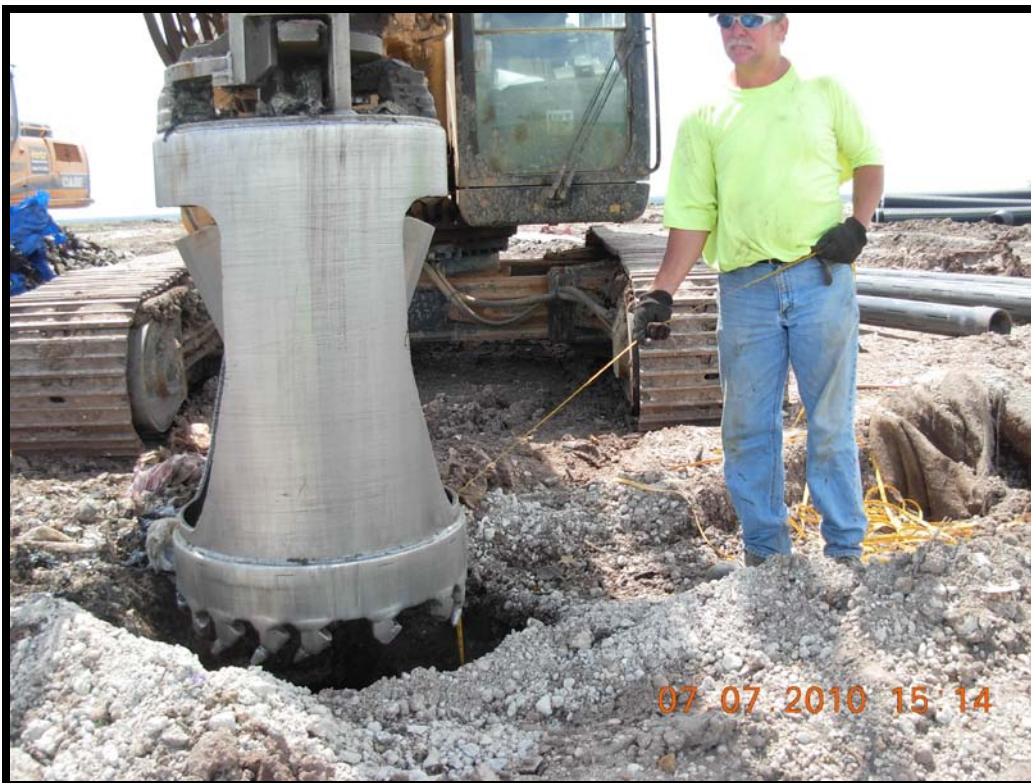
Photograph 10: Measuring bore hole depth at extraction well GW-45.
