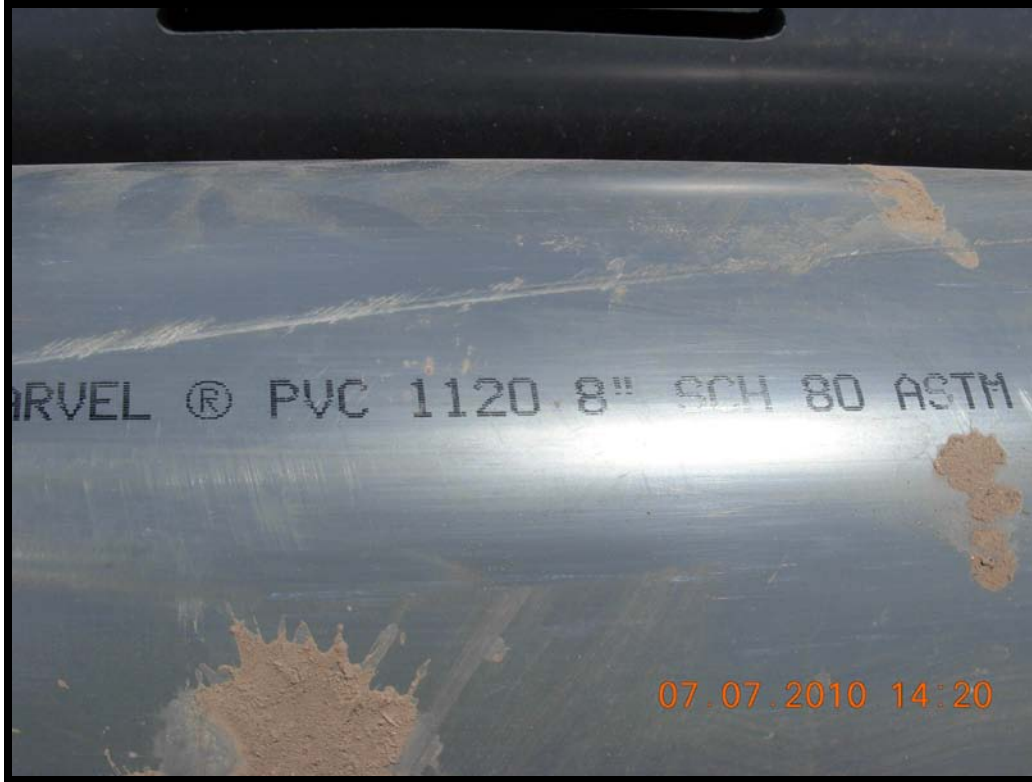
Photograph 7: 8" SCH 80 PVC pipe.
