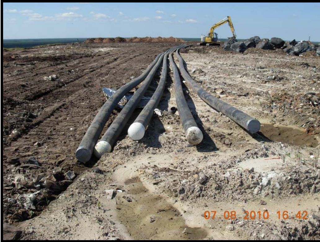
Photograph 13: 6" HDPE SDR 17 lateral strings with end caps.
