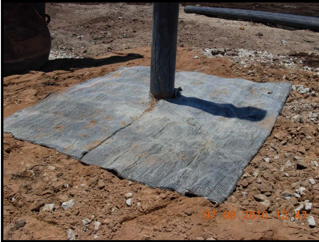
Photograph 23: GCL sheet at extraction well GW-45.
