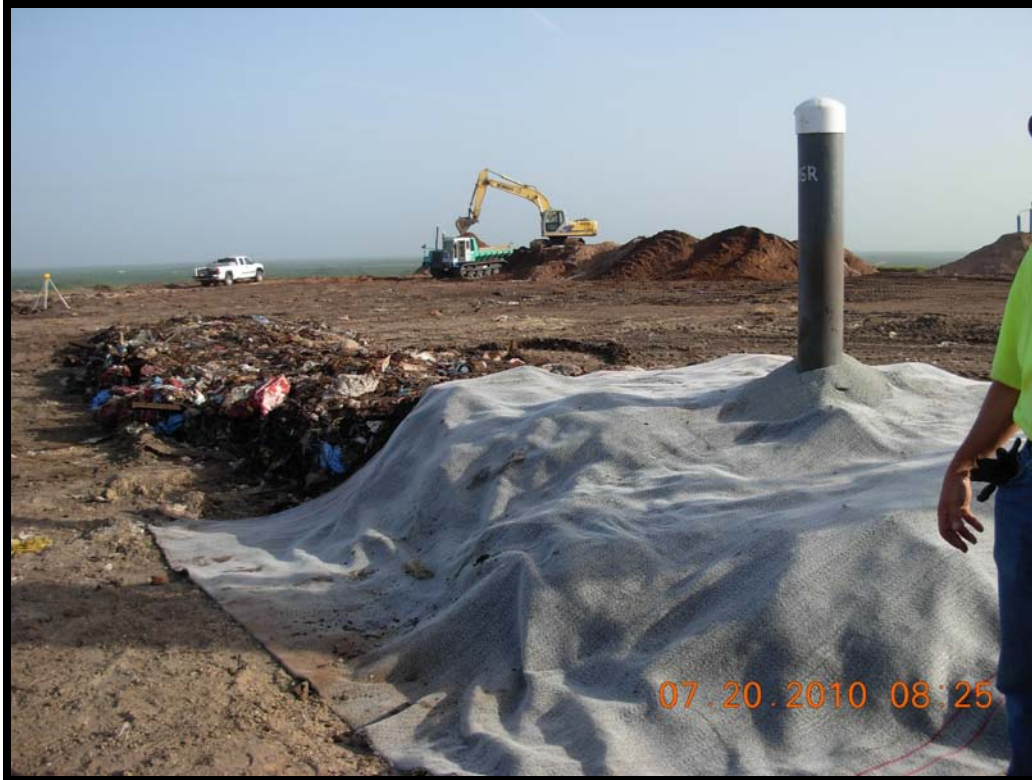
Photograph 51: GCL sheet placed over built-up trash used to maintain a minimum 5 percent slope for the temporarily above ground lateral to GW-15R.
