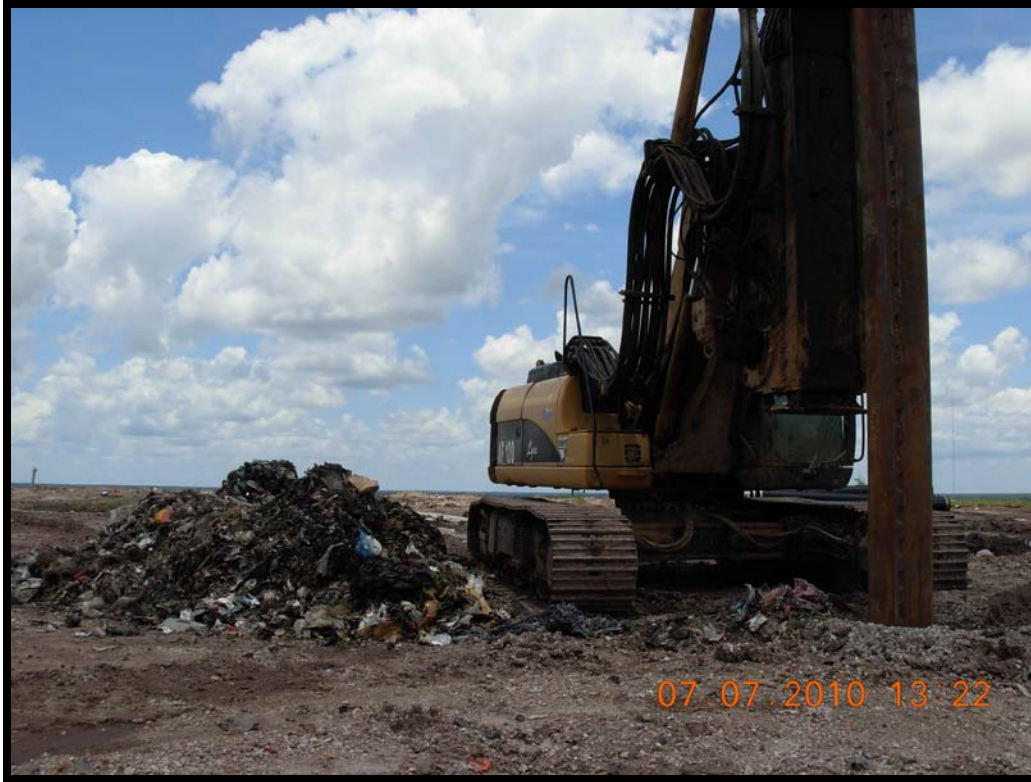
Photograph 9: Drilling extraction well GW-45.
