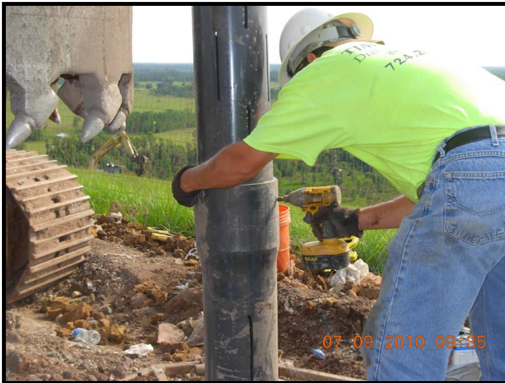
Photograph 26: Lag bolting joints to provided additional support at GW-50.
