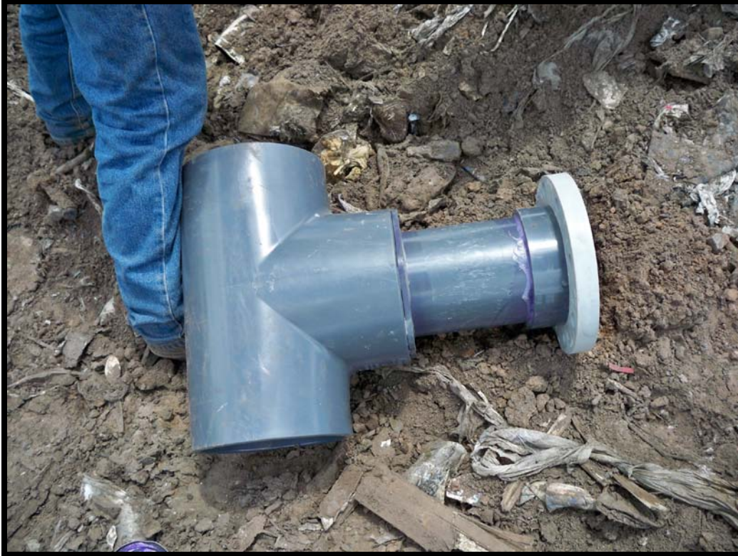
Photograph 61: 8" PVC tee that reduces to 6" with flange to be installed at remote well GW-36.
