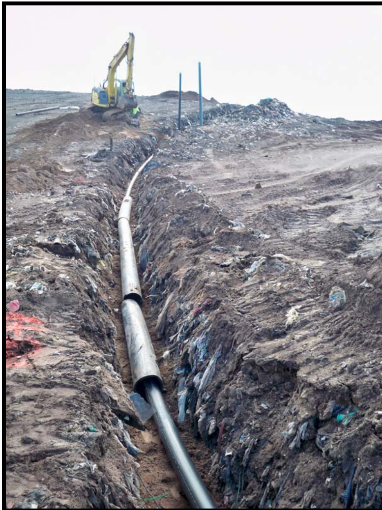
Photograph 66: Looking west, road crossing lateral trench going to GW-54.
