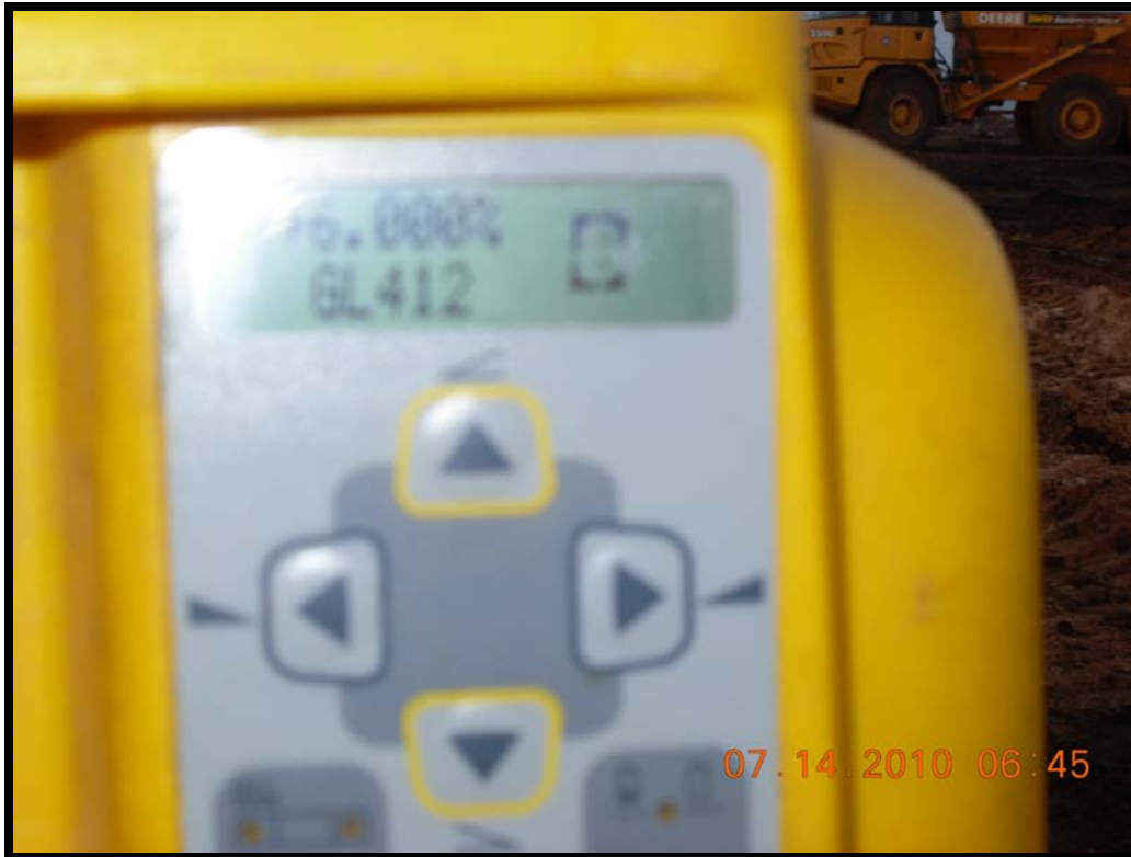
Photograph 38: Survey slope construction laser set at 6% for trenching lateral to GW-40R.
