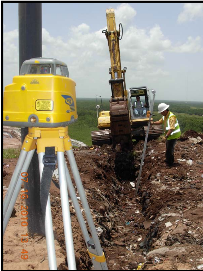
Photograph 43: Survey slope construction laser set at 6% for trenching lateral to GW-18.
