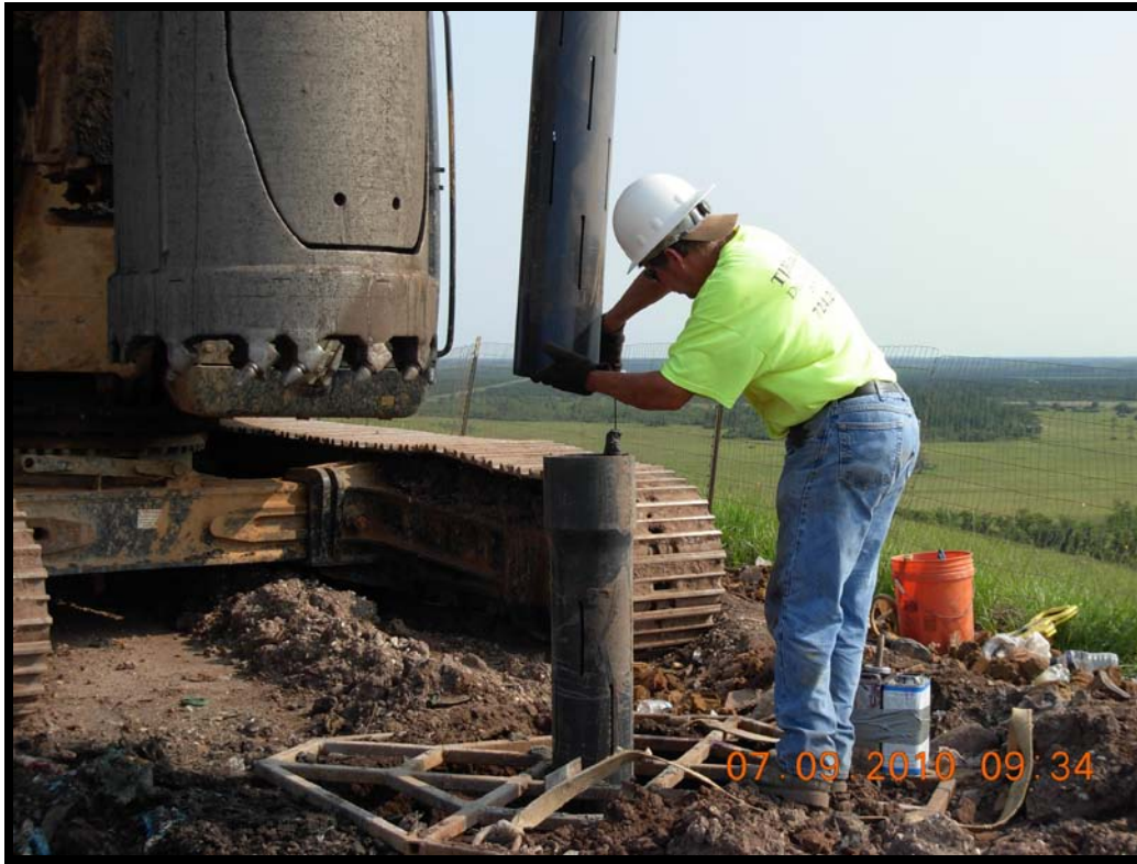
Photograph 25: Applying PVC cement to slotted pipe at GW-50.
