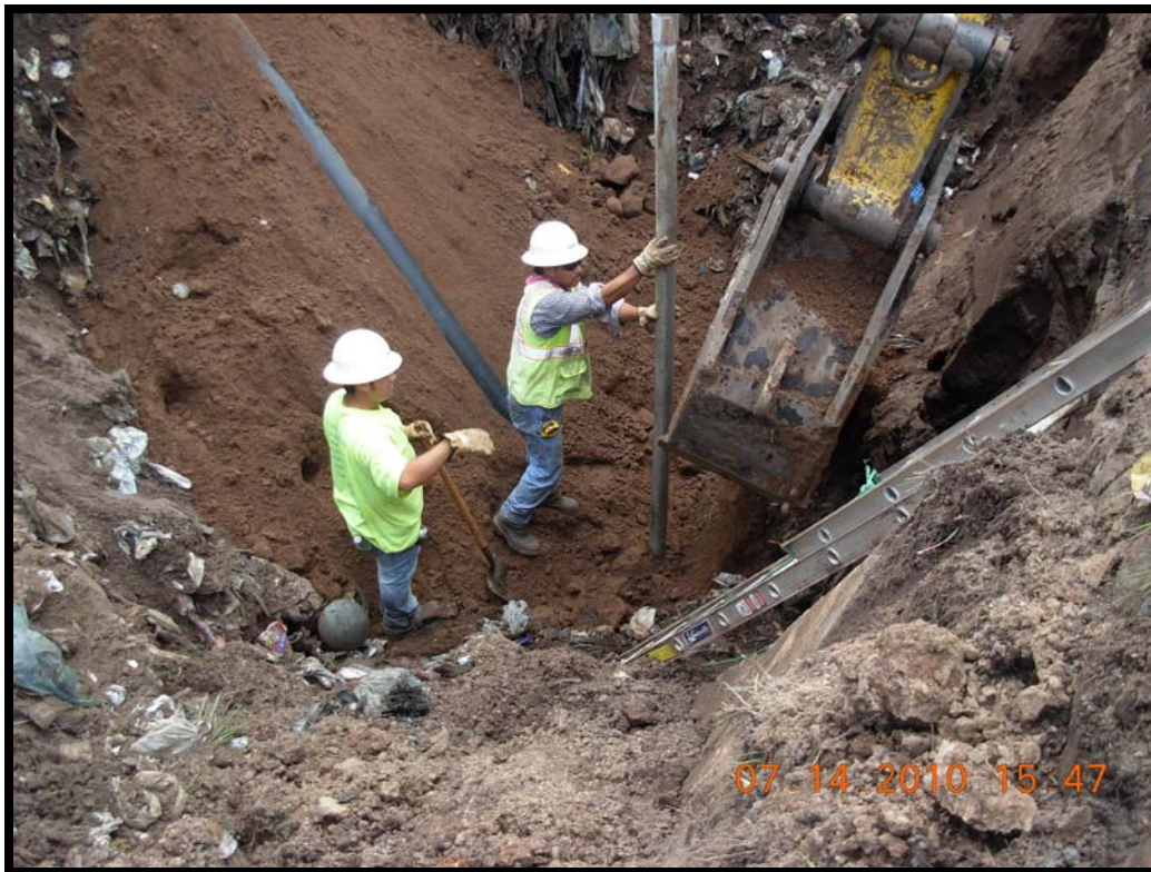
Photograph 41: Placing survey risers on top of lateral tie-in to GW-4R.
