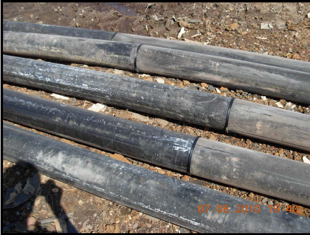
Photograph 15: 6" HDPE SDR 17 lateral hard welds.
