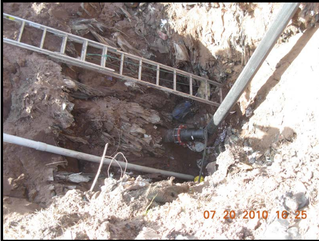
Photograph 49: Extraction well GW-27 lateral tie-in to existing 8" HDPE flange. 8" reduces to 6".
