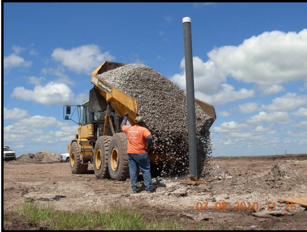
Photograph 17: Backfilling extraction well GW-45 with stone.
