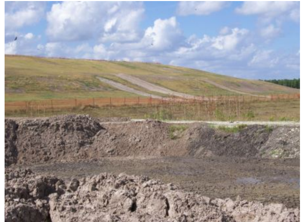
Filled Area of Dewatering Ditch
