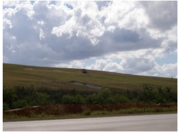
Closed Class I Erosion Repair
