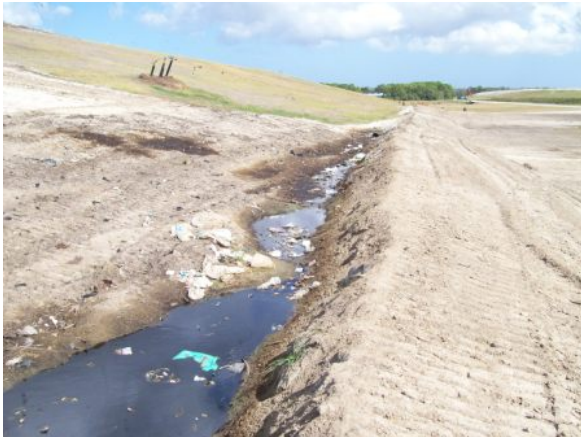
South Side Slope Leachate Seepage
