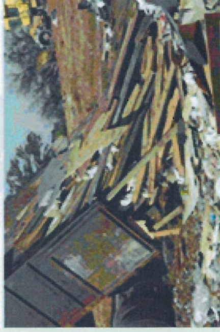
Top: Loads from the demolition of outdoor structures will typically contain CCA-treated wood. Pole at the upper left is treated. Complete recovery of untreated wood from this pile will likely require testing in addition to visual separation.
