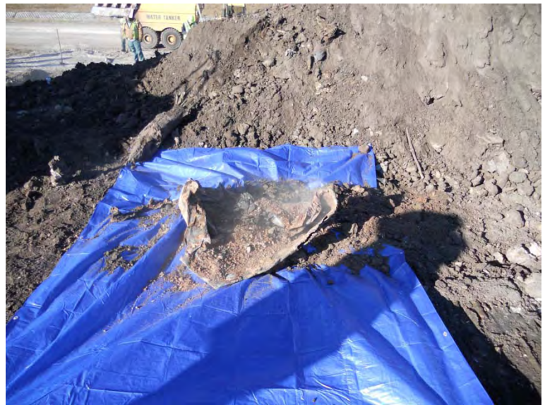
12/9/2010 Excavated waste placed on tarpaulin for identification DSCN0011.JPG
