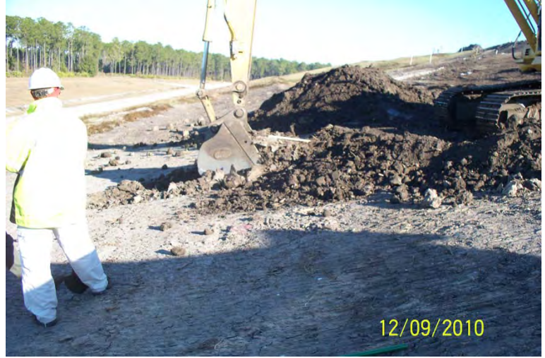
12/9/2010 Excavating to determine the condition of the bottom liner 100_0570.JPG
