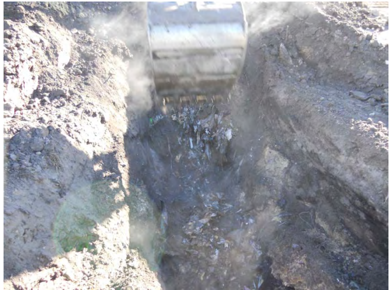
12/9/2010 Unburned / unaffected waste being excavated DSCN0023.JPG
