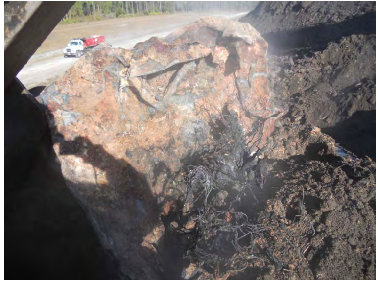
12/9/2010 Charred, burnt waste excavated from location of subsurface fire DSCN0010.JPG
