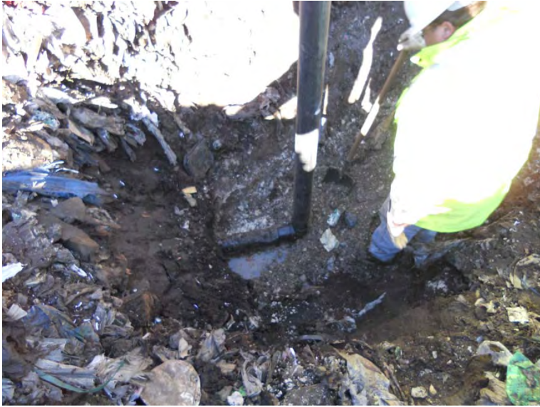
12/7/2010 Installing the 90' replacement lateral and abandoning the compromised lateral DSCN0002.JPG
