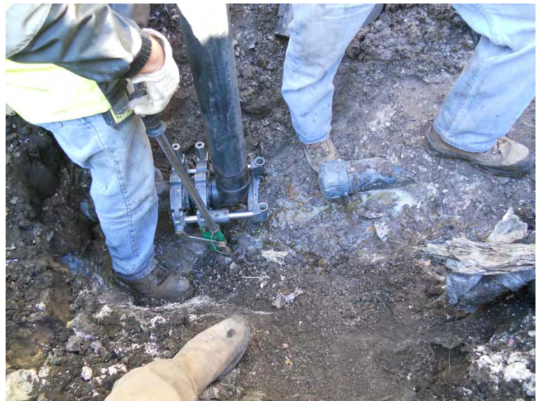
12/7/2010 Cutting, capping the lateral DSCN0001.JPG
