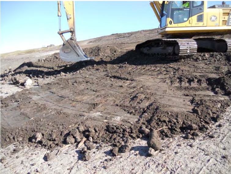
12/9/2010 Excavation backfilled and compacted DSCN0035.JPG
