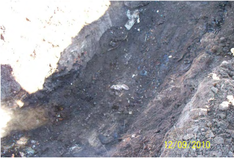
12/9/2010 Protective san layer exposed; no sign of damage apparent. 100_0586.JPG
