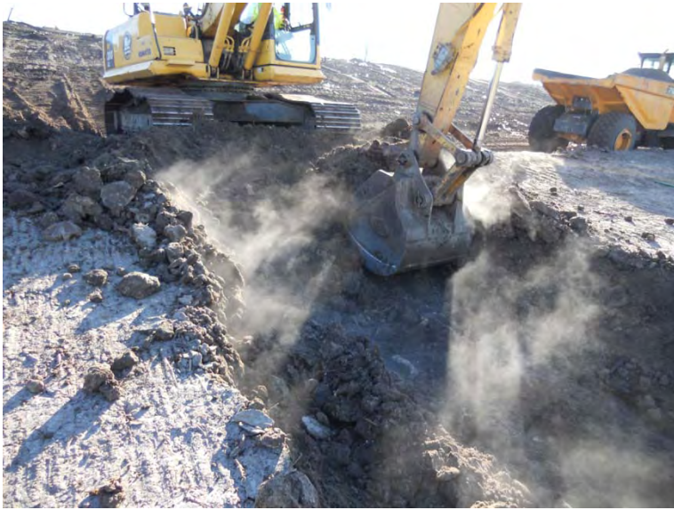
12/9/2010 Excavation to determine the condition of bottom liner being performed DSCN0004.JPG
