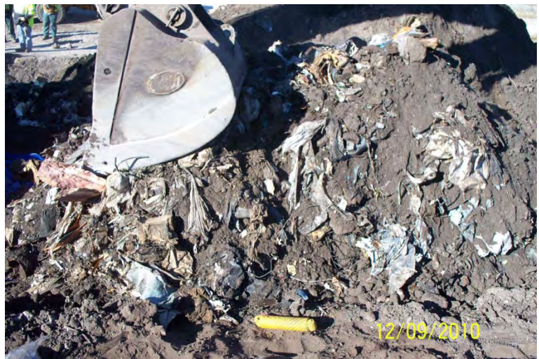
12/9/2010 Unburned waste removed from excavation 100_0585.JPG
