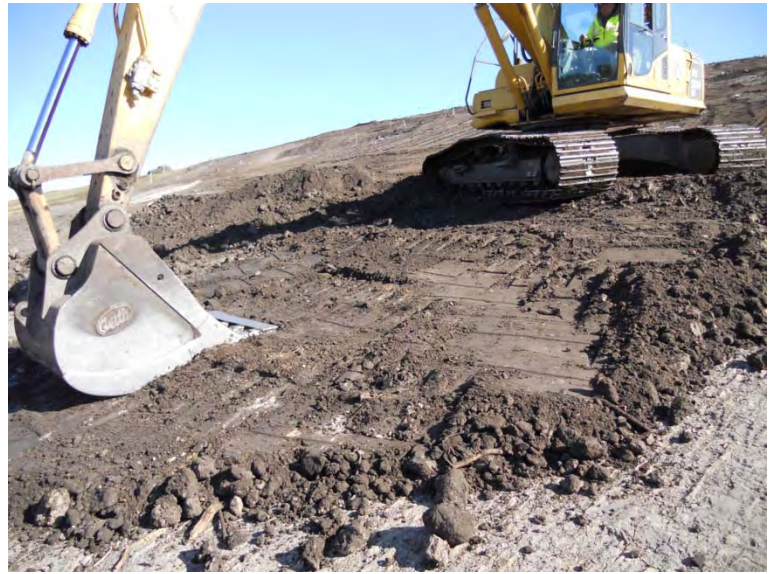
12/9/2010 Excavation backfilled and compacted DSCN0034.JPG
