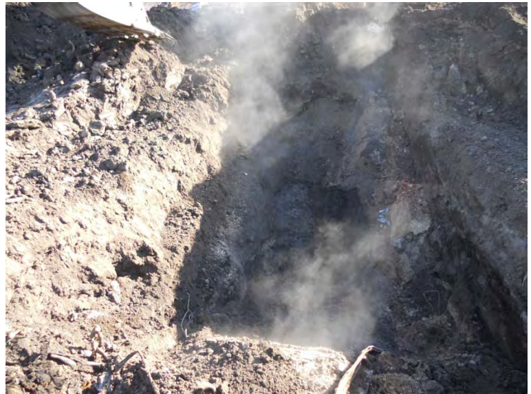
12/9/2010 Exposed sand layer; little sign of being affected by high combustion temps DSCN0018.JPG
